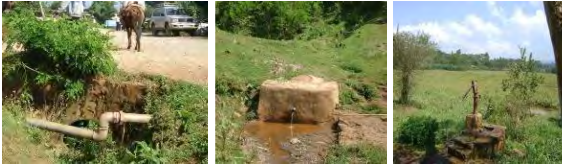
Photo 7-1: Some potentially affected water supply schemes – Water supply pipeline crossing the road at ~km 19.5 at Sheki town (left), protected spring source at km 22.60, 10m RHS below the road (middle) and hand pump at ~km 7.20, 10m LHS located at edge of a wetland spot (right)
