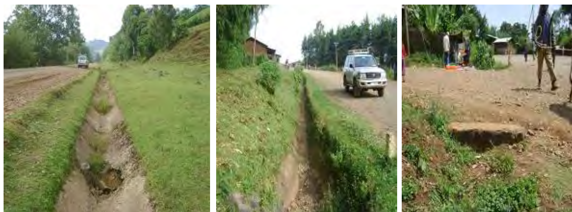
Photo 5-2: A view of well-functioning concrete lined roadside ditches at km 34 (left) and km 21 (middle), and a completely silted up pipe culvert at km 20 at junction to internal road (right)
