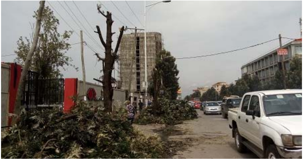
Figure 8-1: An example of cutting roadside trees that contact with electric lines and cause power outages.
