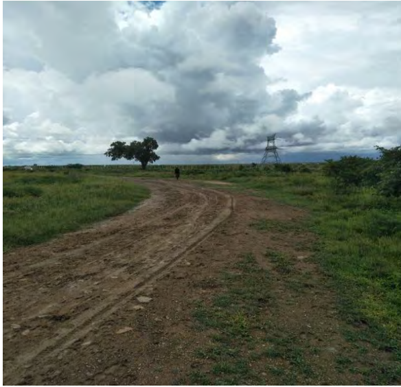
Beginning of the transmission line at Mariakani Sub - Station
