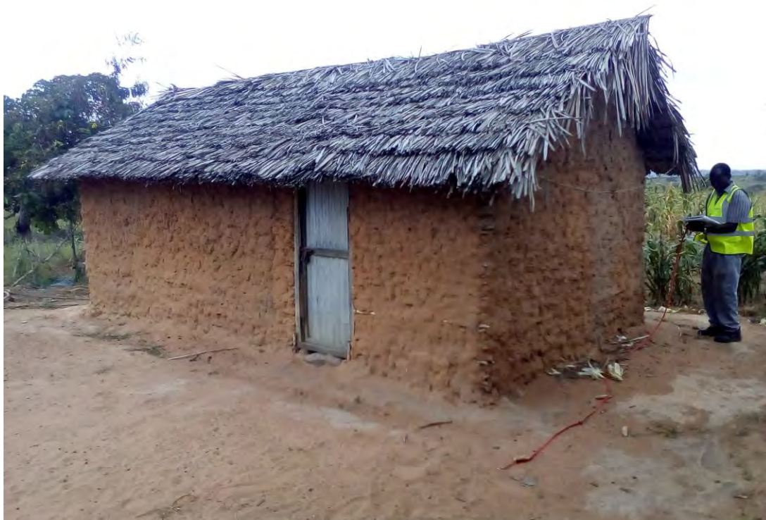
Photo 1: Inspection of Affected Structure in Progress - July 2017
