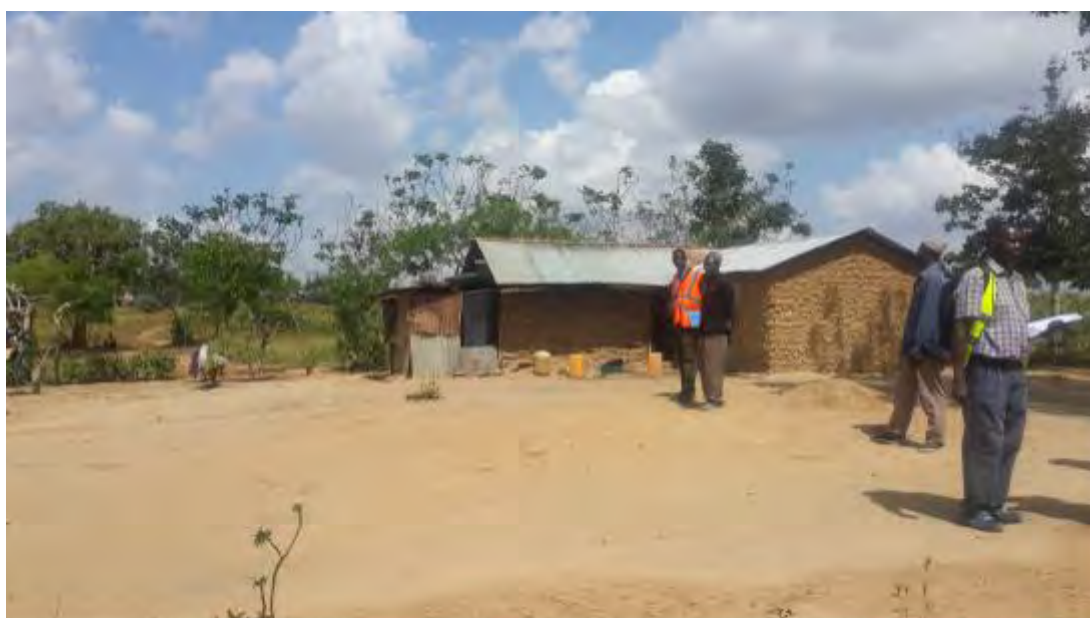
Plate 6: Housing Structures Affected by the TL Corridor – July 2017
