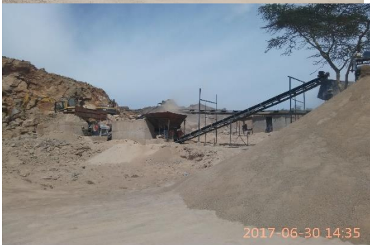
Photograph 1-2: Quarry at km 128.850
