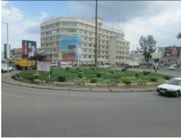
Photograph 4-21: First Roundabout – Gate House Roundabout
