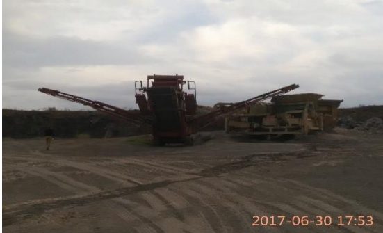
Photograph 1-4: Borrow Area at km 124.000
