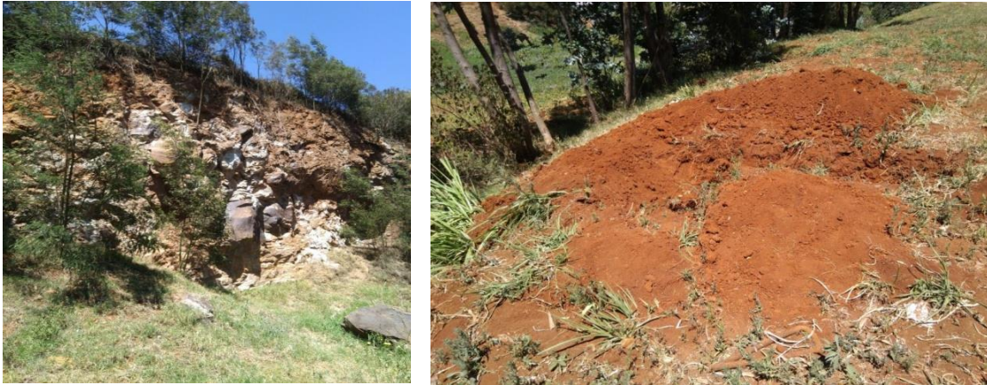
Figure 4-2. Rocks and Soils in Mutarakwa Road Corridor
