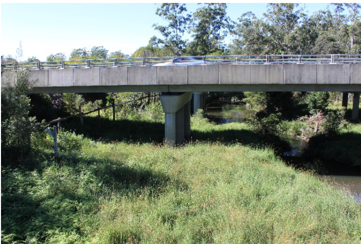
Figure 4.4. (Left) Example of a well-designed bridge underpass that is open, with a natural substrate and continuous vegetation compared to a poorly designed bridge underpass (right) with minimal space on both sides of the waterway and over-use of large rocks for erosion control that hinders the movement of many species. Photos Rodney van der Ree, WSP.
