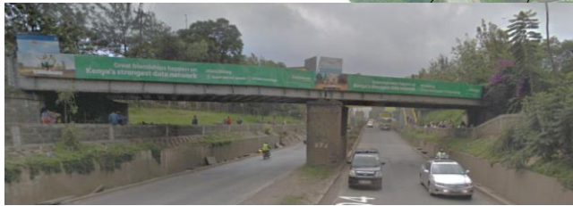
Railway bridge maintained
