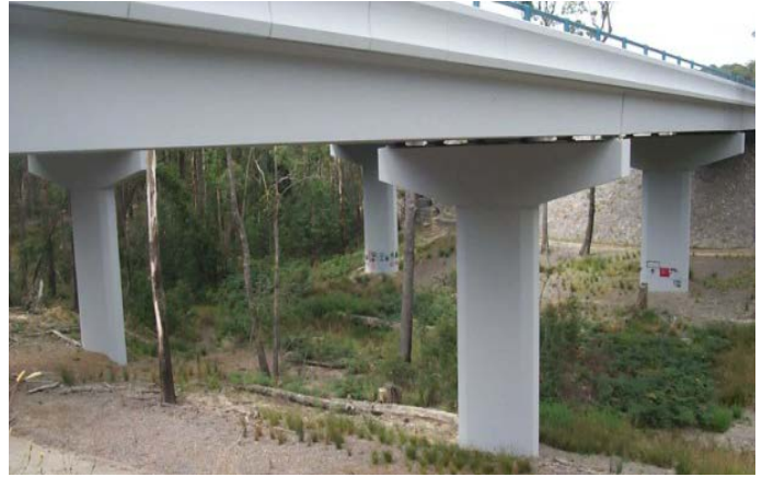
Figure 4.3. The Slaty Creek Bridge on the Calder Freeway in south-east Australia was designed to be higher and longer than required simply for drainage, to encourage wildlife movement. In this example, the vegetation has been planted underneath the structures, and tall trees retained between the two carriageways. This is an example of a very large bridge – most do not need to be this large. Photos Rodney van der Ree, WSP.
