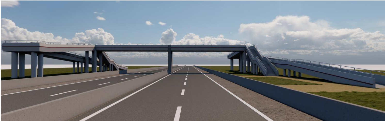
Footbridge with stairs and ramps
