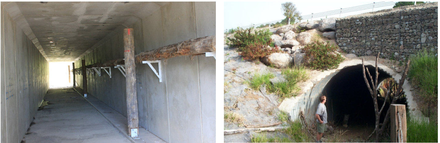
Figure 4.6. (Left) Interior of a recently constructed wildlife culvert, with a timber rail for scansorial and arboreal species. (Right) large arch culvert with logs and branches providing furniture for arboreal wildlife.
