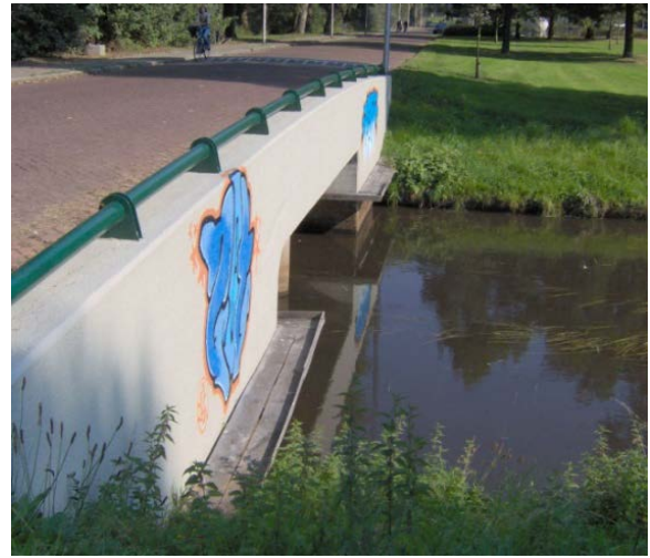
Figure 4.9. Example of strategies that provide dry passage if the culvert contains standing or flowing water. Note that the concrete ledge and timbershelf in the left photo are still to be connected back to the adjacent habitat. Photos by Rodney van der Ree WSP.
