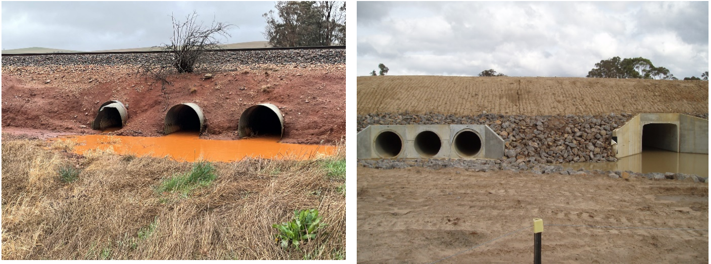
Figure 4.7. Poor drainage and ponding can reduce the effectiveness of all types of culverts and they must be carefully designed, constructed and managed to effectively enable both uses. Photos (left) Rodney van der Ree WSP and (right) Scott Watson VicRoads.
