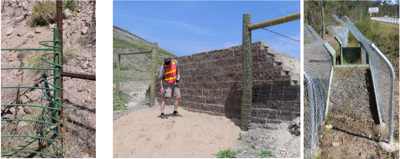
Figure 4.16. Example of one-way gates (left) and jumpouts (middle) from the USA and Pacific Hwy NSW (right) to allow animals that breach wildlife fencing and find themselves trapped between the fence and the highway to escape. A limitation of one-way gates is that they can become stuck in the ‘open’ or ‘closed’ positions and become ineffective. Jump-outs must be designed and tested for the target and non-target species to ensure they are unable to climb up and into the highway reservation. Photos Rodney van der Ree WSP.
