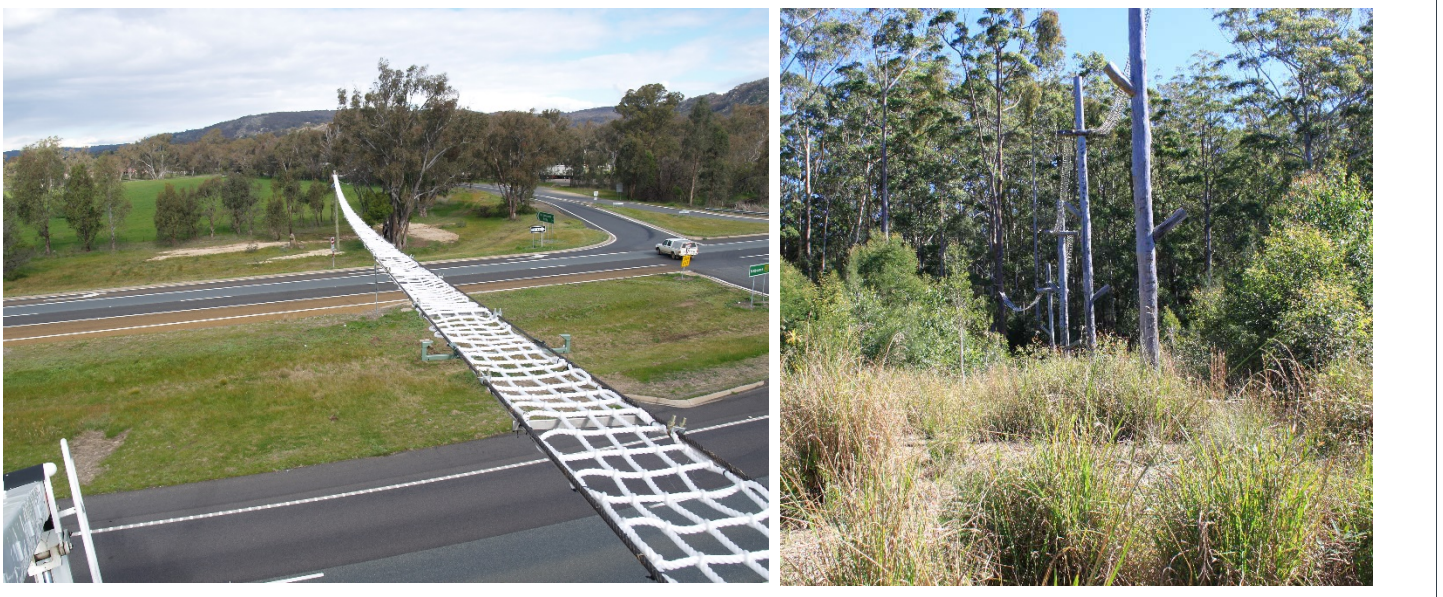
Figure 4.10. Canopy rope bridge across a highway (left) and on top of a land bridge (right), both in Australia
