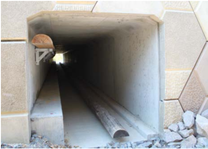
Figure 4.9. Example of strategies that provide dry passage if the culvert contains standing or flowing water. Note that the concrete ledge and timbershelf in the left photo are still to be connected back to the adjacent habitat. Photos by Rodney van der Ree WSP.
