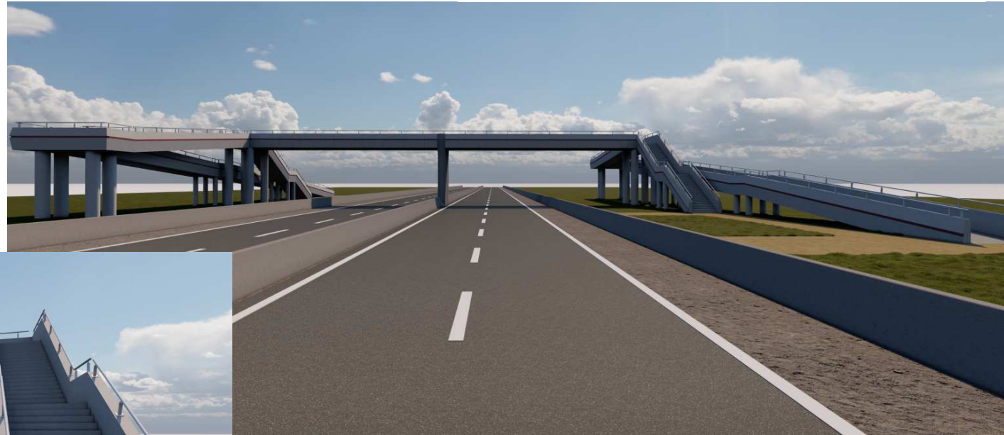
Footbridge with stairs and ramps
