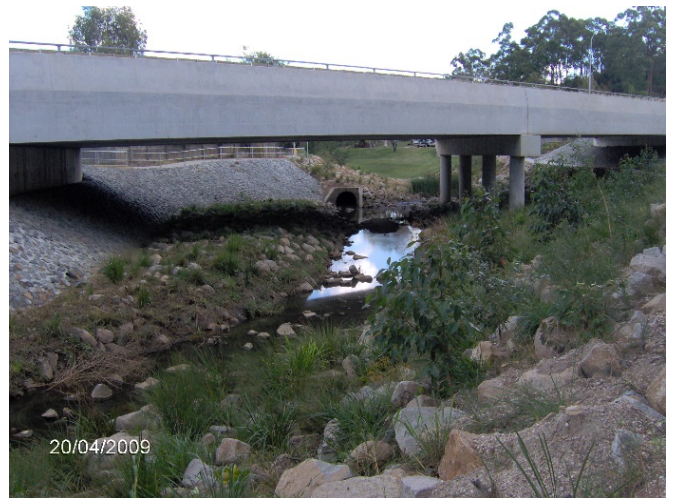
Figure 4.4. (Left) Example of a well-designed bridge underpass that is open, with a natural substrate and continuous vegetation compared to a poorly designed bridge underpass (right) with minimal space on both sides of the waterway and over-use of large rocks for erosion control that hinders the movement of many species. Photos Rodney van der Ree, WSP.
