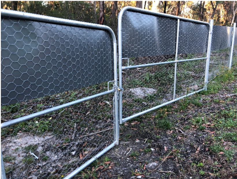
Figure 4.14. Care must be taken to avoid gaps under wildlife fencing, especially at gates and where fencing is attached to crossing structures. Photo Josie Stokes WSP.
