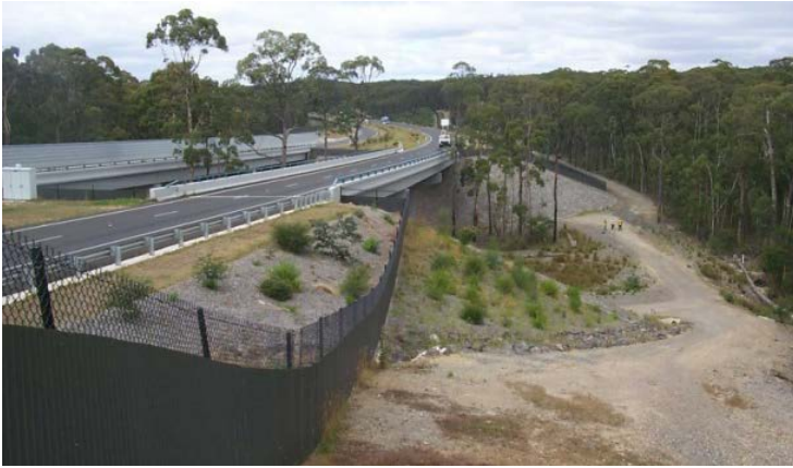
Figure 4.3. The Slaty Creek Bridge on the Calder Freeway in south-east Australia was designed to be higher and longer than required simply for drainage, to encourage wildlife movement. In this example, the vegetation has been planted underneath the structures, and tall trees retained between the two carriageways. This is an example of a very large bridge – most do not need to be this large. Photos Rodney van der Ree, WSP.
