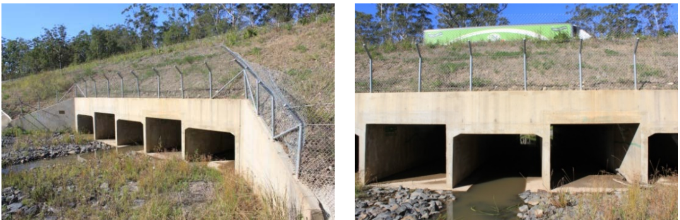
Figure 4.8. Example of multi-cell culverts on the Pacific Highway NSW where the middle cell is designed to take water flow year-round, with the outer cells remaining dry except during flood events. Photos Rodney van der Ree WSP.
