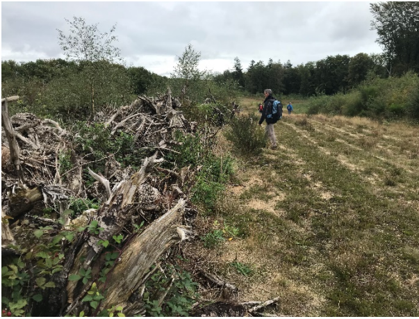
Figure 4.2. View on the top of land bridges that are 50 – 70 m wide in The Netherlands and France, showing rows and piles of tree stumps and shrubs within grassy areas which provide habitat and 'furniture' for a range of different species and enable views across the bridge.
