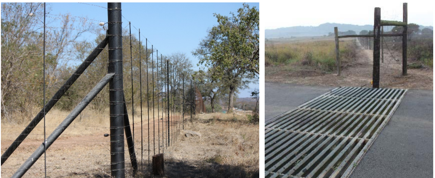
Figure 4.13. Electric fencing with wire mesh at the base and dug into the ground (left) is a standard and effective approach to controlling the movement of wildlife in East Africa, and will be installed in continuous lengths in Marula and Soysambu and in shorter
