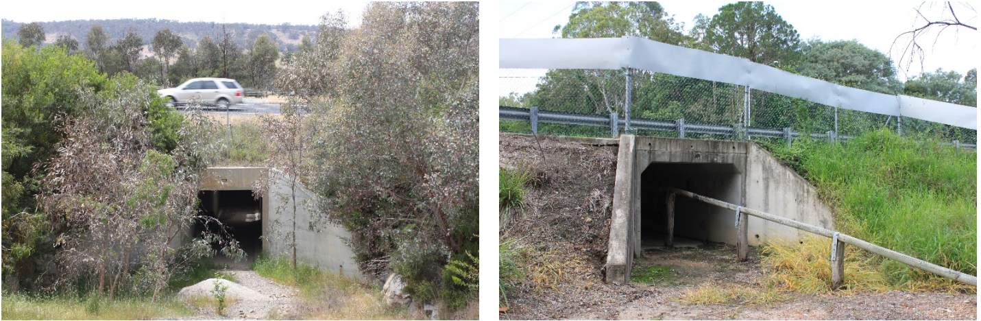
Figure 4.5. Dedicated 3 m x 2 m (left) and 2 m x 2 m (right) culverts for wildlife. Culverts are smaller than open span bridges and present as a 'tunnel' to wildlife and are likely less effective than bridge underpasses for open-country species.
