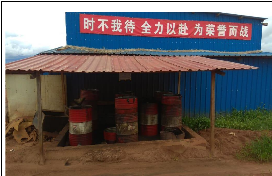
Storage area with spill containment base
