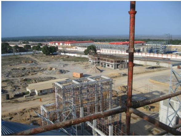
Nacala Industrial Zone (Flour milling factory under construction)
