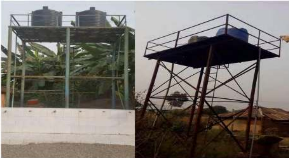
Plate 4.51: Borehole facility @ Sowunmi and Ajade communities respectively
