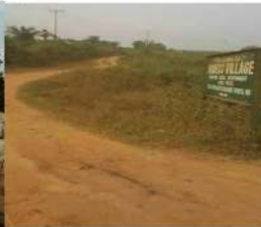
Plate 4.56: Papalanto-Soderu Road (Earth road).
