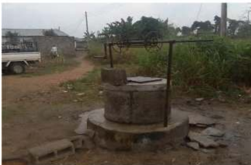
Plate 4.52: Community water well facility in Olorunsogo Community
