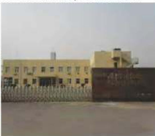
Plate 4.48: Olorunsogo Power Plant Phase I
