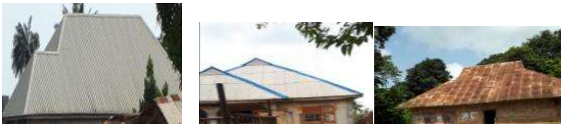
Aluminum roofing in Bandu | Corrugated iron sheet in Olaoparun | Asbestos in Igbele
