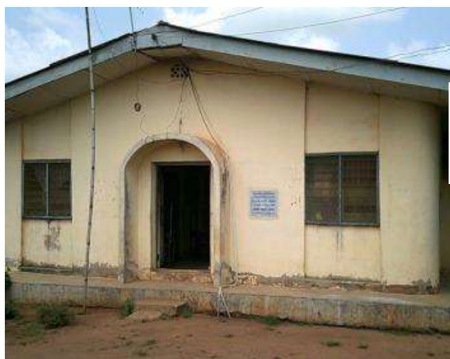
Plate 4.26: A Primary Health Centre in Ajegunle (Ado Odo Ota LGA)
