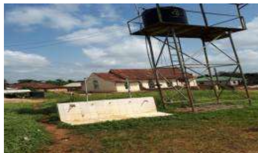
Plate 4.24: Borehole Facility in Ekundayo
