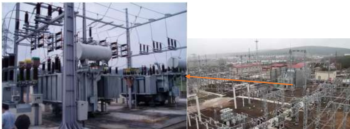
Figure 2.3 A Typical AIS Substation (with transformers zoomed in)
