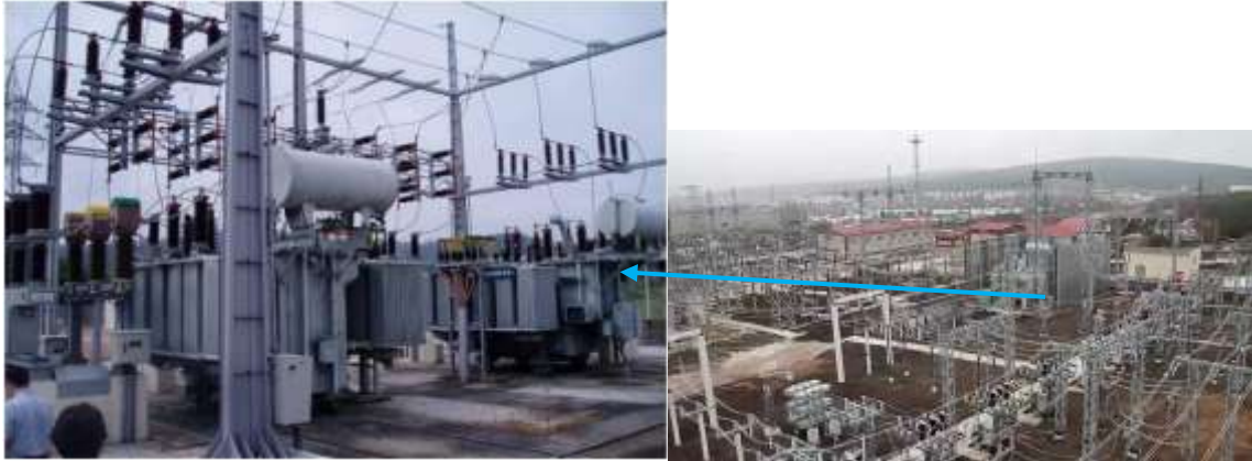
Figure 3.12A Typical AIS Substation (with transformers zoomed in)
