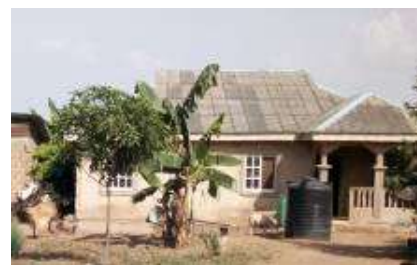
concrete in Berese
