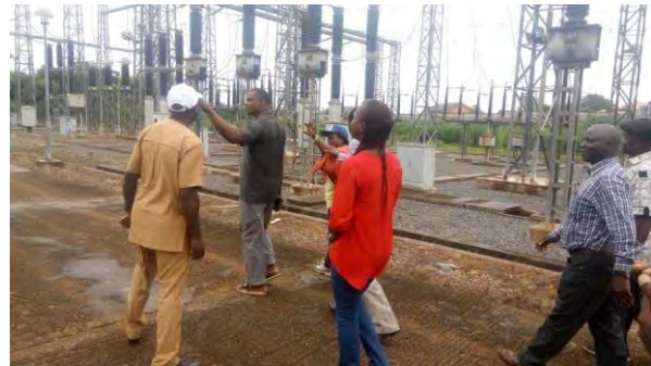
At Ikeja West Substation
