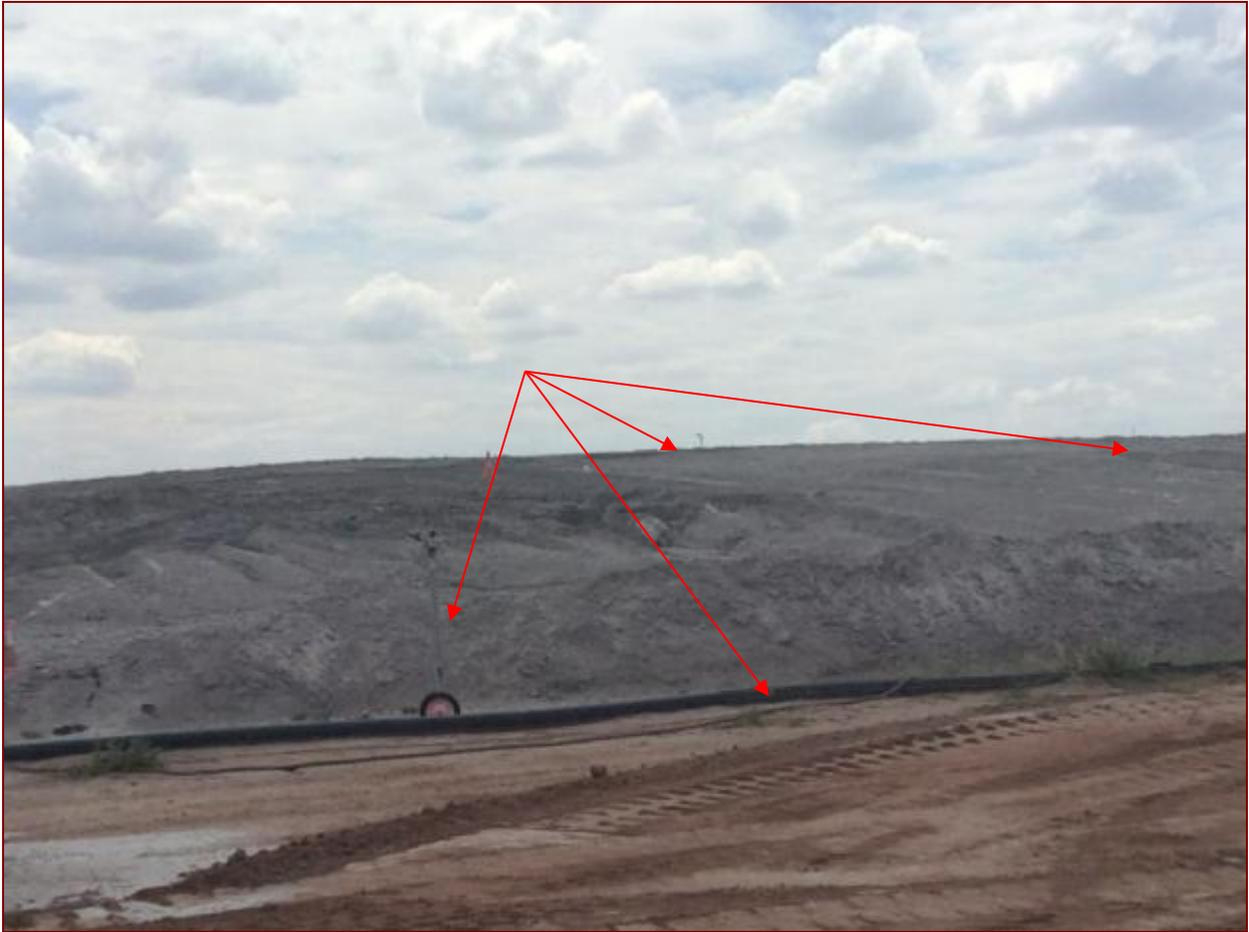
*Figure 46- Sprinkler system developed to suppress dust*
