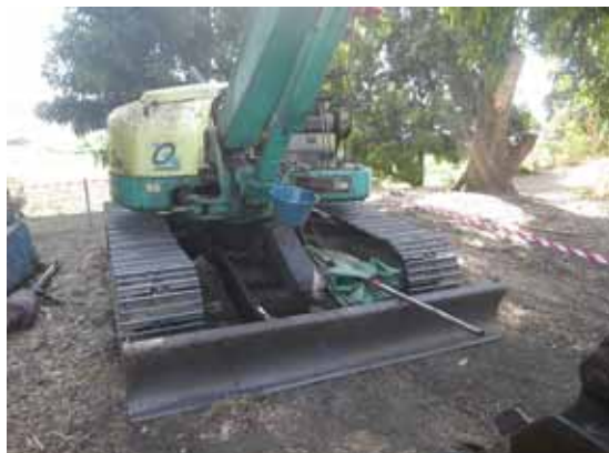
Rig is carried by mini crawler crane (Note the width is 2m only)
