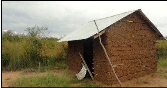
Photo 1.1: Typical house type close to the proposed project site.
