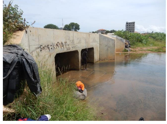
No.19 橋梁の現況
