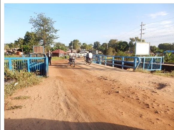
No.21 橋梁の現況
