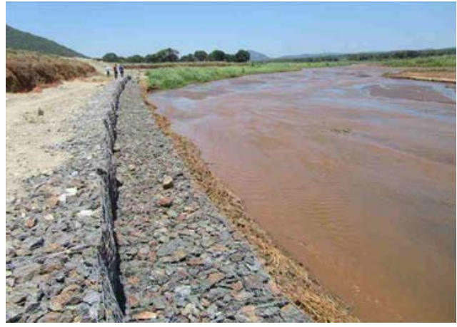
Plate 82: Gambion protected river embankment at Site Km 315.1
