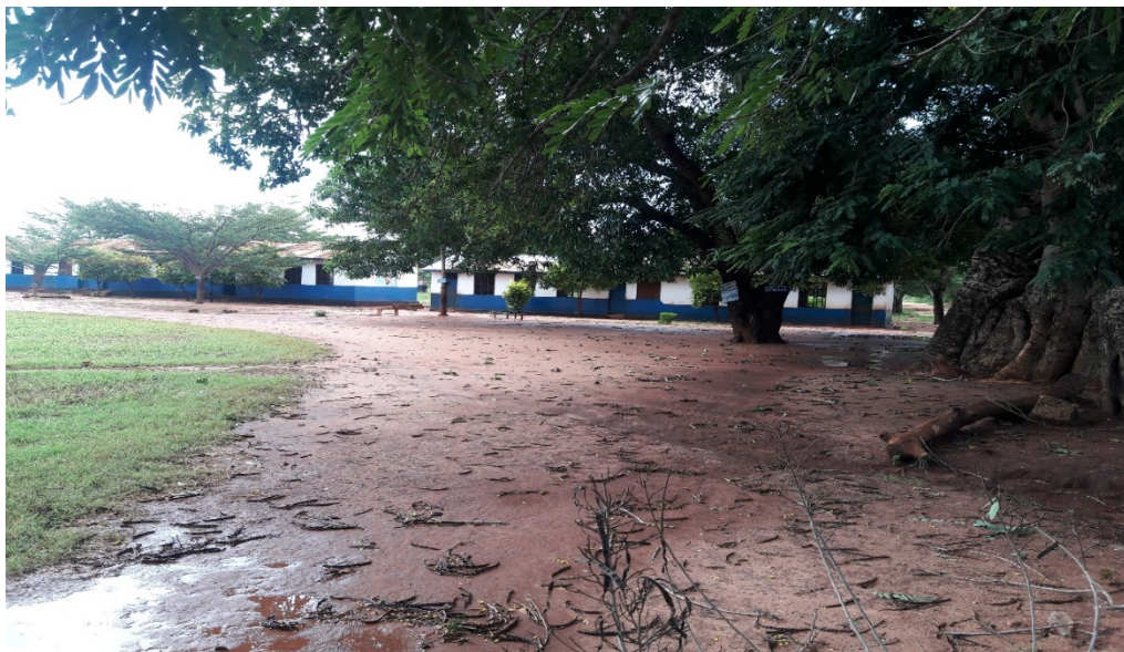
Figure 4-31 Namgogoli primary school in Mtwara rural district
