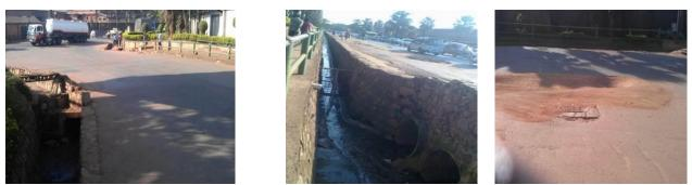
Photo 5-7: The drainage of the area. The pothole shown is probably as a result of some water ponding on the road surface as opposed to running into the drain.
