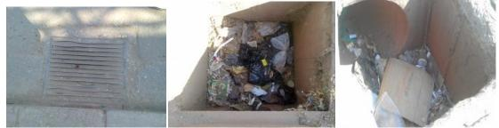
Photo 5-3: Blocked Drains and Waterways around the Clock Tower Area (August 2013) The figures above show blocked drains and water ways around clock tower area.
