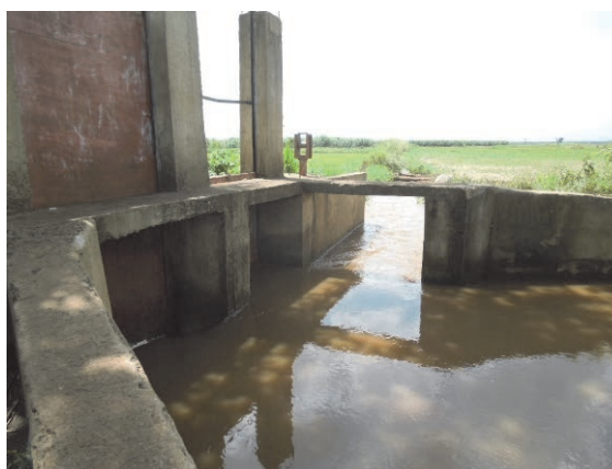
Intake along the Atari River
