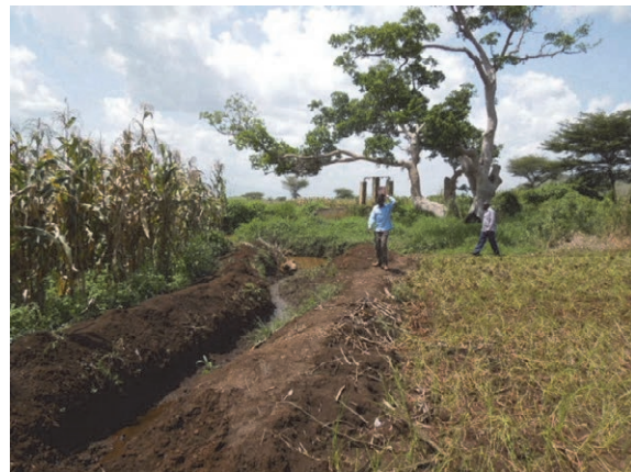
Diversion of Atari Left Bank
