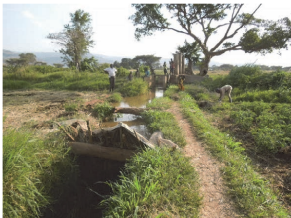
Diversion Weir at Right Bank Main Canal
