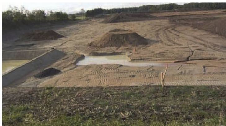
Photo-2 Temporary Sedimentation Pond
