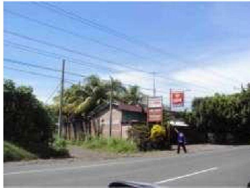
Photograph No. VI.43. View of the road to El Delirio (RN17) at the final point of the Project
