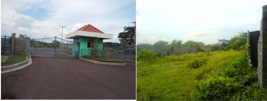
Photograph No. VI.33. View of urbanized land use in this project section, housing project Anagil Afife and abandoned half-built houses in housing development Los Angeles.
