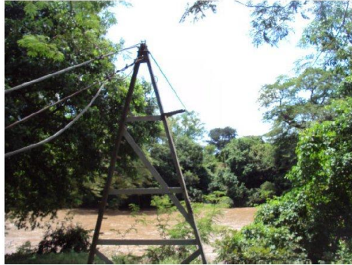
Photograph No. VI.29. Crossing by cable over the river near station 9+150
