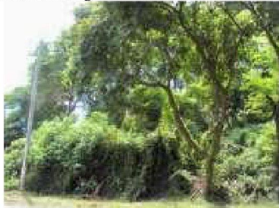
Photograph No. IX. 1. View of the almost verticle cut-off in the proposed protected área, which keeps stable due to the rocks present
