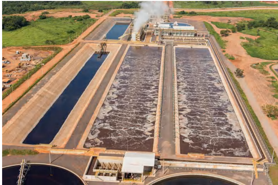
Figure 30 –Aeration tanks
