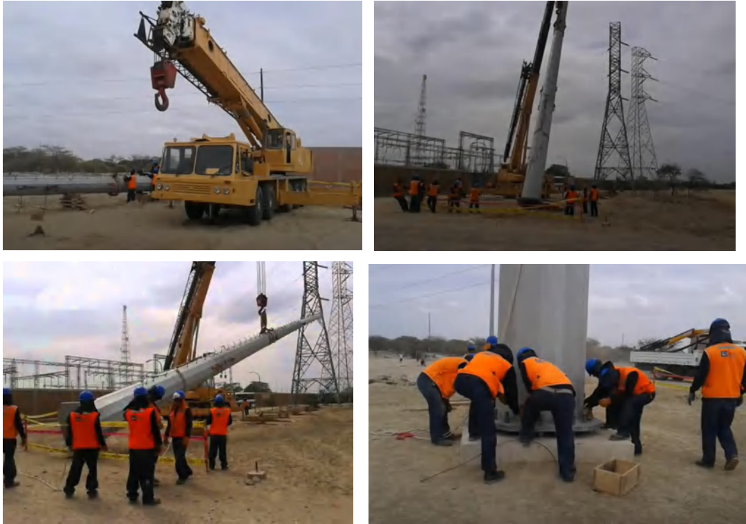
Figure 49 – Example of assembly of the towers
