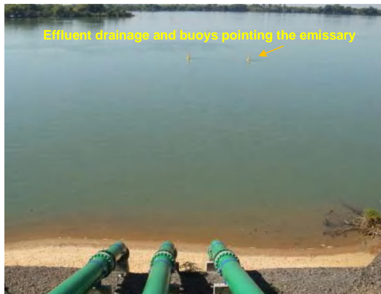
Figure 32 – Effluents emissary pipeline
