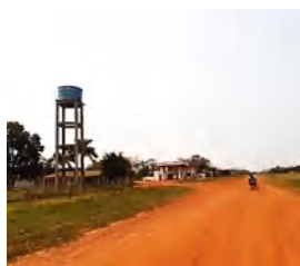
Water System, Center of Puentesíño
