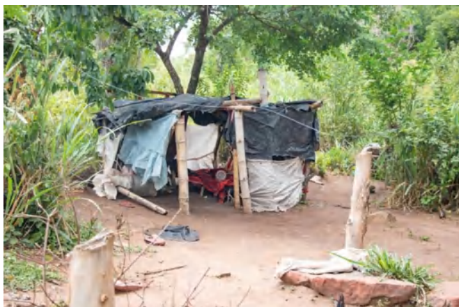
Photo: makeshift house with palm trunks and plastic.
