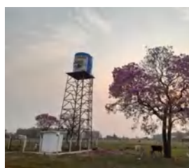
Water System, Paso Barreto
