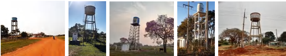
Water System, Center of Puentesíño
