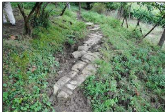
Figure E-41: Stonework in Zestafoni
