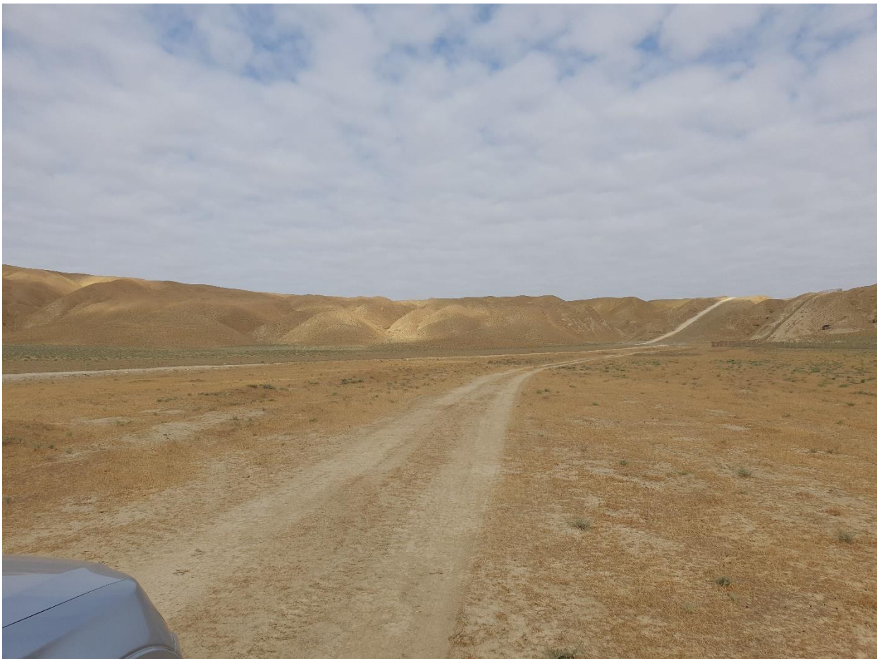
Figure 1-4: Example section of the existing track to be used for the new access road
