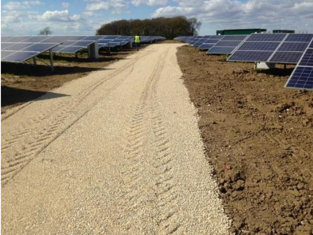
Figure 2-14: Typical internal access track
