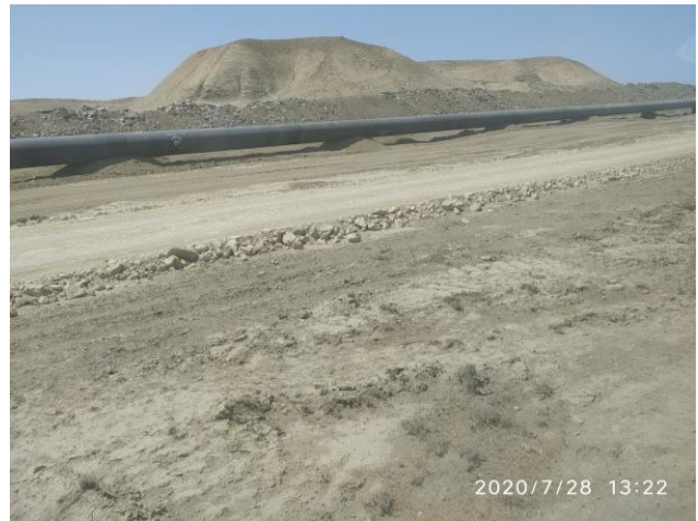
Photo 6. Route of underground gas pipeline under construction
