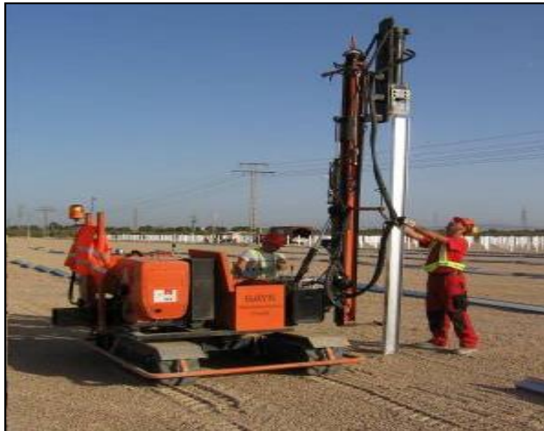
Figure 2-9: Hydraulic Driving Machine for Installing Piles
