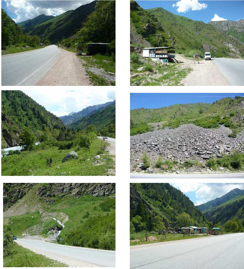
Figure 1.3 Condition at objective area
