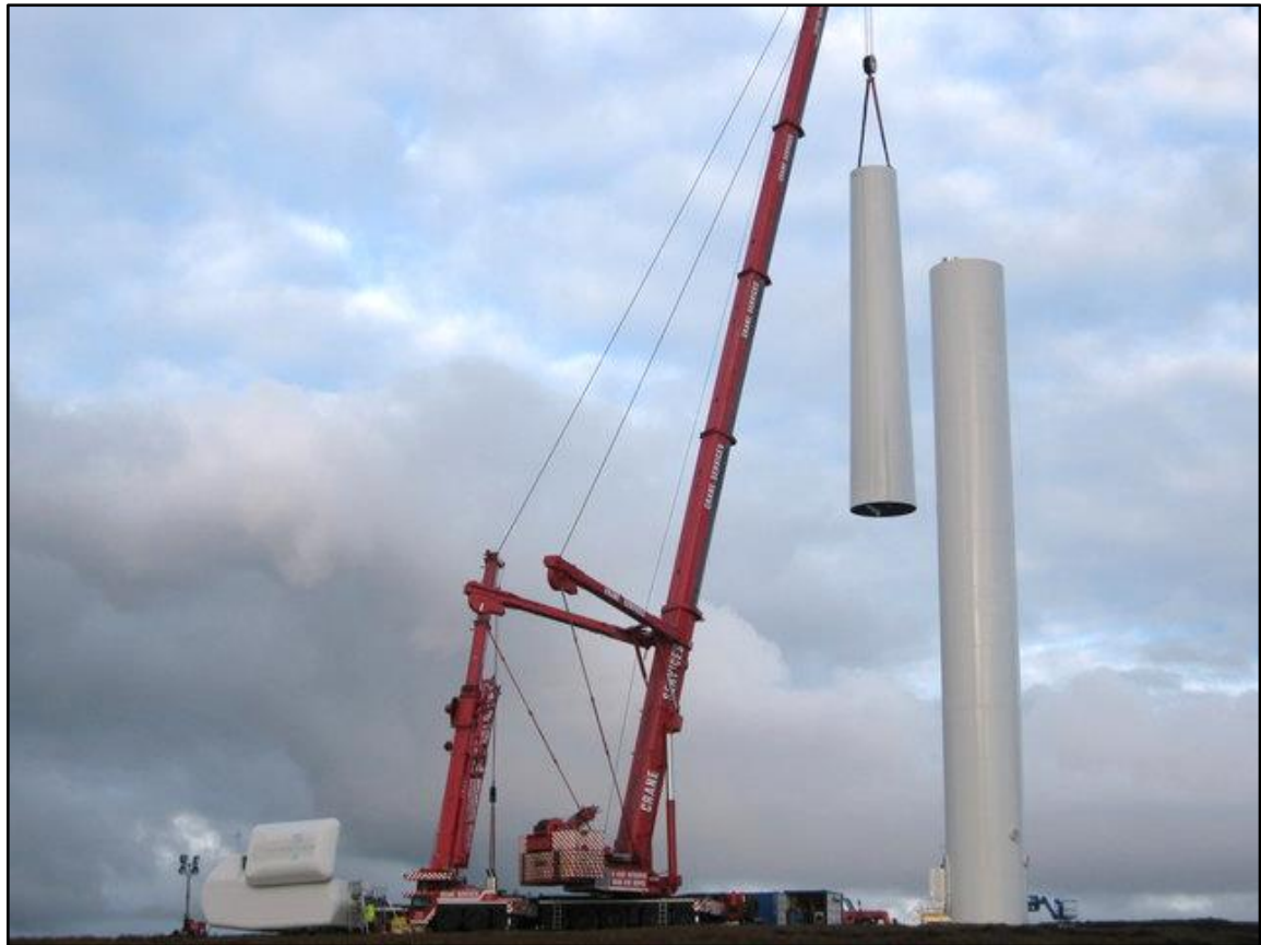
Figure 2-10: Typical WTG tower
