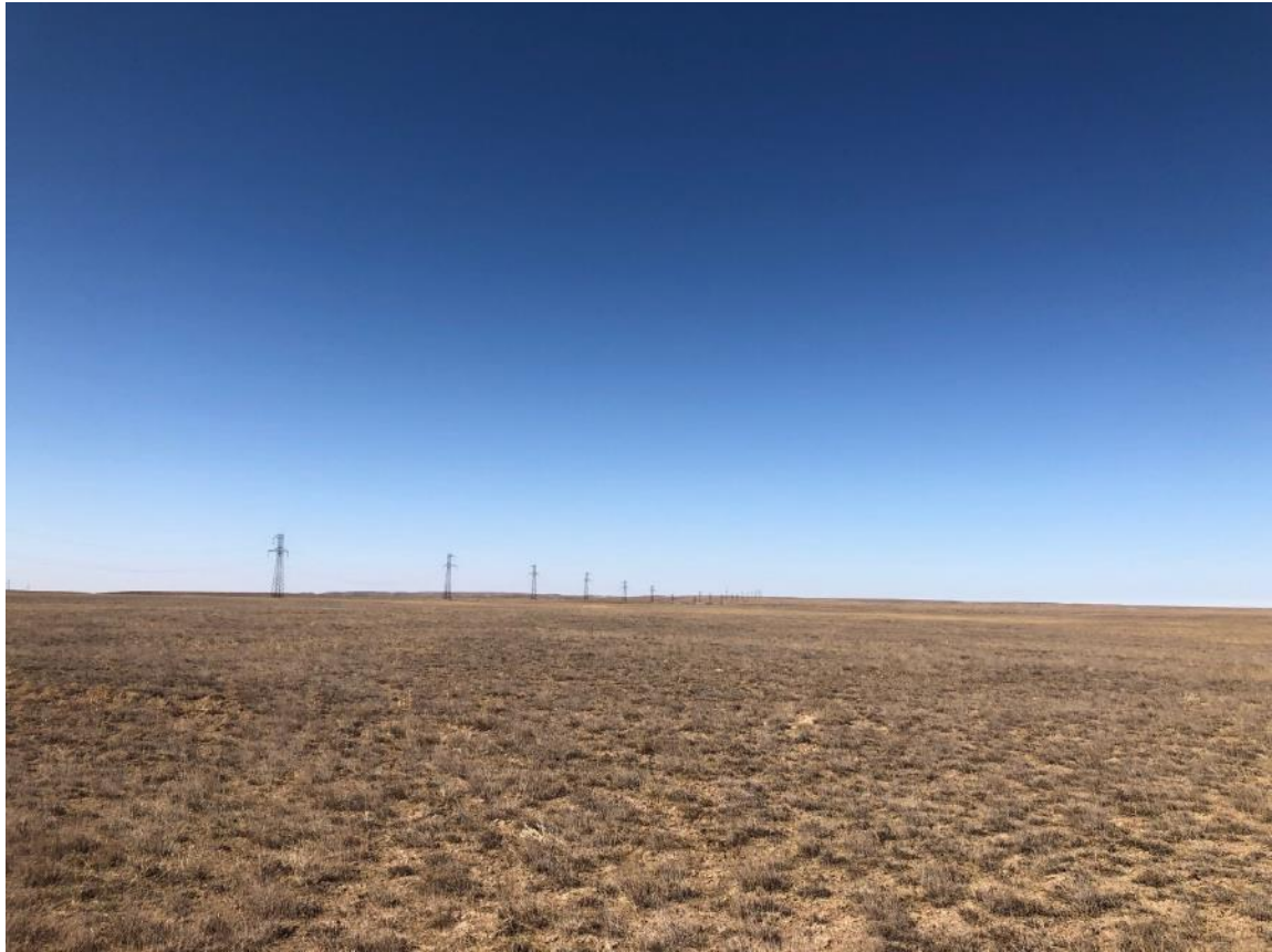
Figure 2-2: Western area of the Project site
