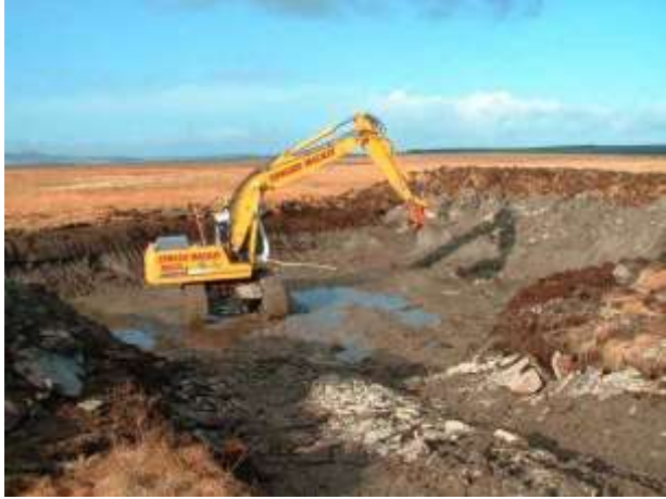
Step 1 – Digging the foundation
