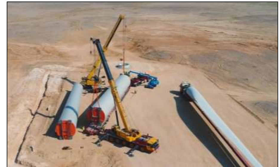
Construction of a wind turbine
