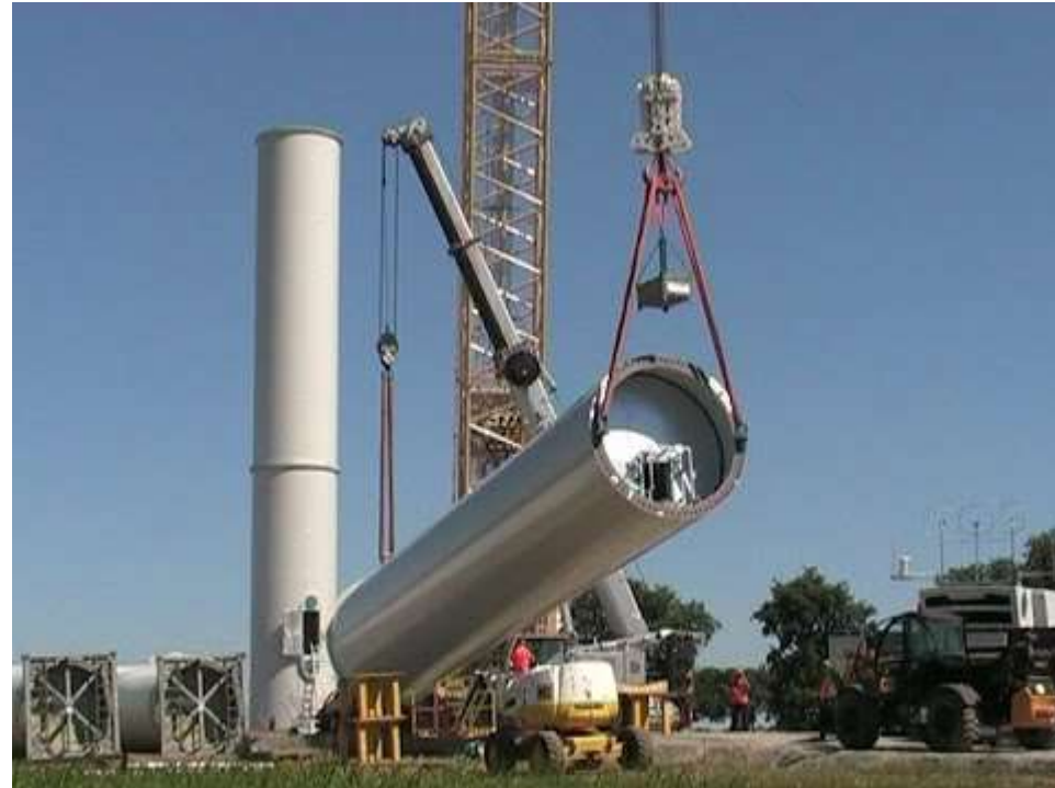
Step 5 – Using cranes to construct the tower
