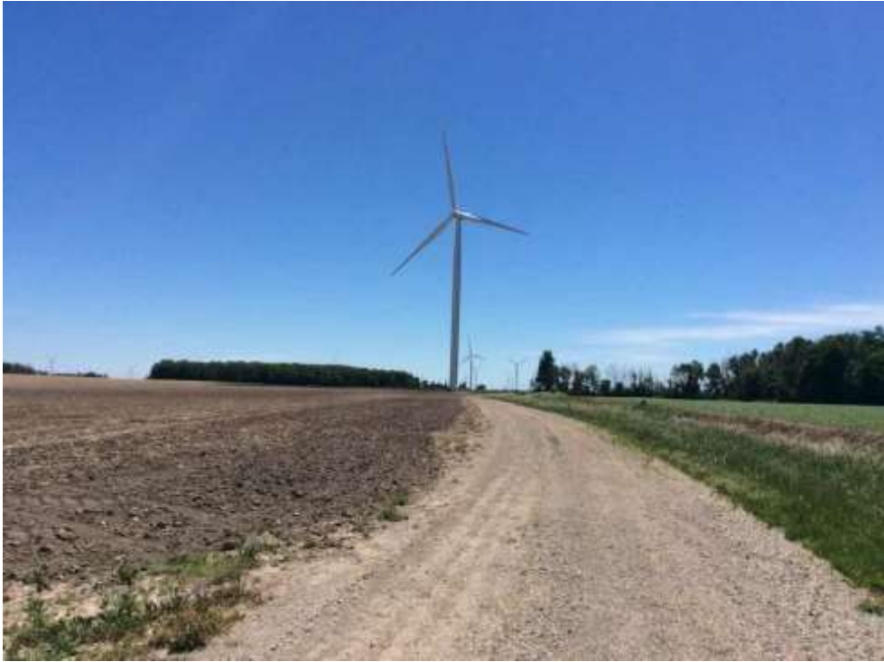
Internal road construction
