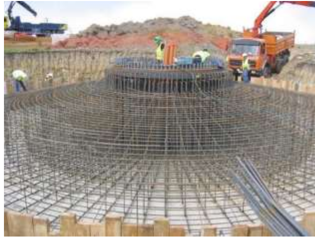
Step 2 – Adding concrete and steel
