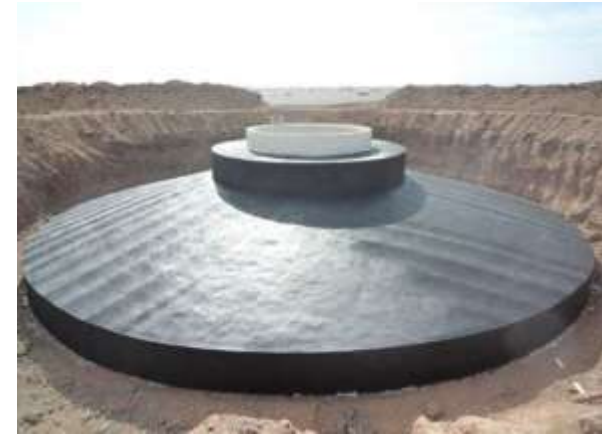
Step 3 – Finishing the foundation
