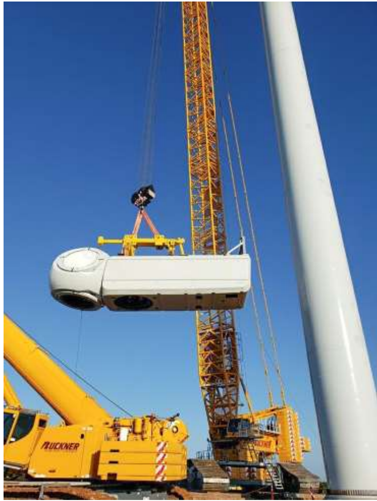
Step 6 – Using cranes to attach the nacelle
