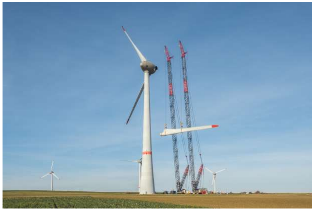
Step 7 – Using cranes to connect the blades
