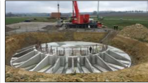
Installation of a foundation base
