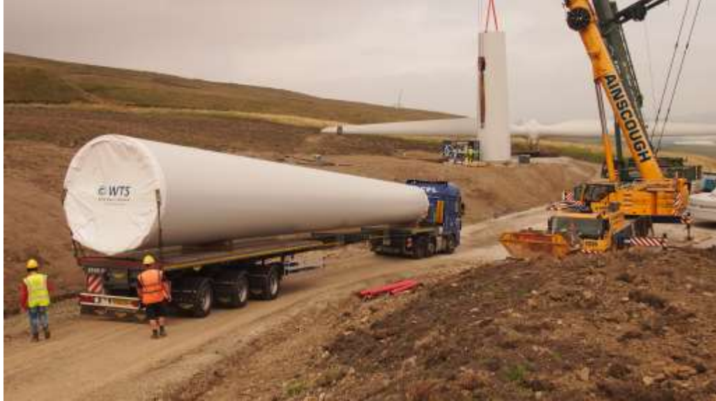
Step 4 – Transporting the components to the foundation
