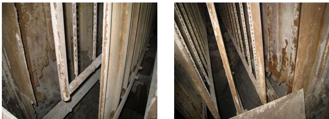
Fig.4.2-25 #4 ESP Inner Parts
