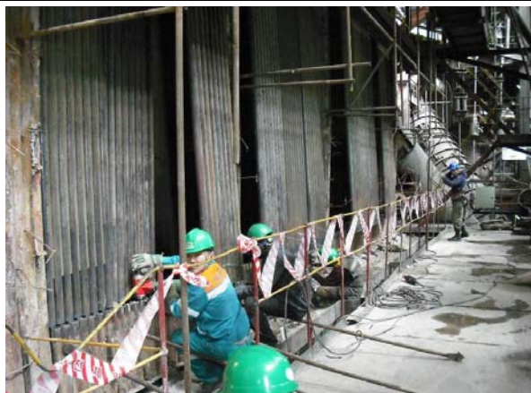
Fig.4.2-27 Replacement of Boiler Water Wall
