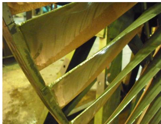
Fig.4.2-17 LP Last Blade after Repair
