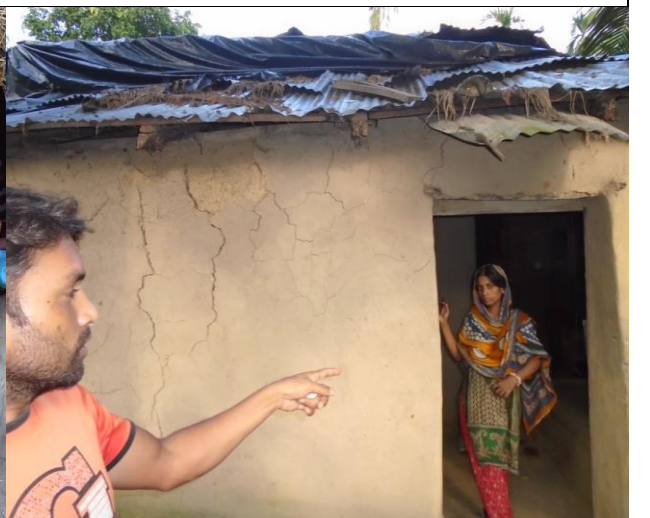
Photo of tin shed Housing structure
