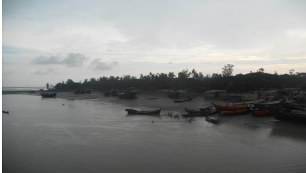
View of proposed alignment and Rajghat Bridge area
