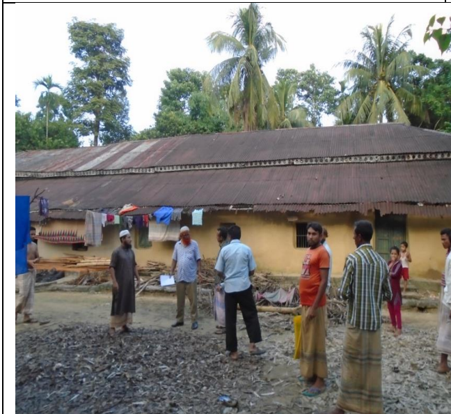
Photo of Semi pucca tin shed with mud wall housing structure
