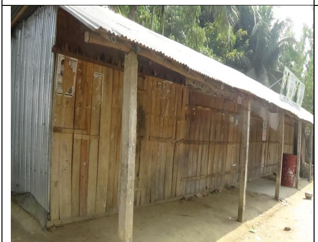
Photo of tin shed shop structure
