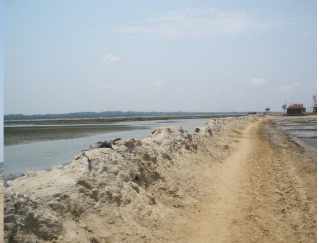
Existing Condition of the Embankment
