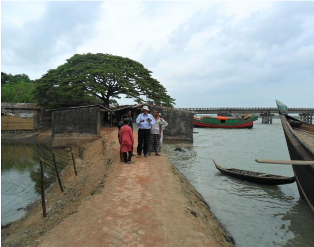
Rajghat Bridge on Koheli River starting point of proposed embankment cum road
