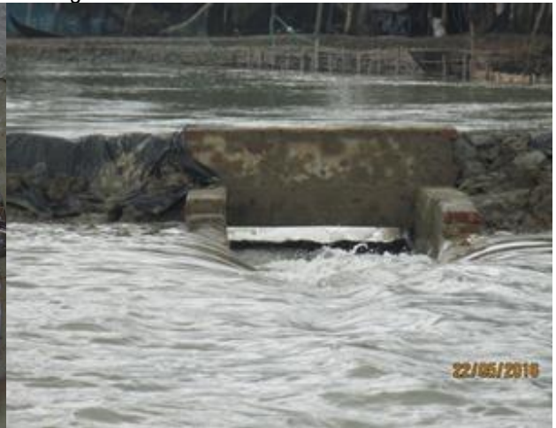
Drainage System in the project area
