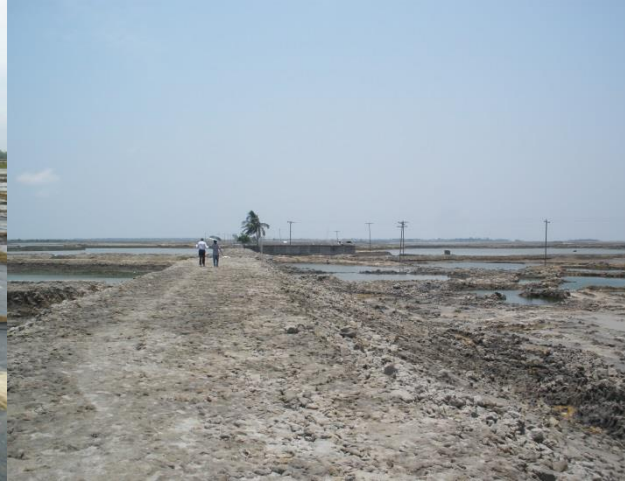
Existing Embankment Condition
