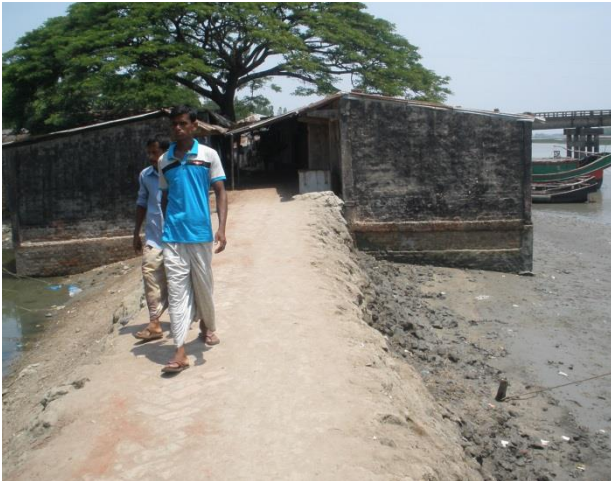
Shops at the Rajghat Point of the proposed embankment cum road
