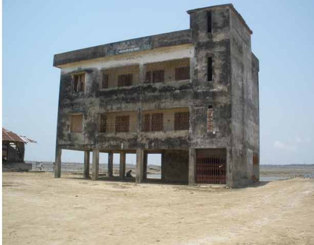
Abundant Cyclone Shelter in the Proposed Road area
