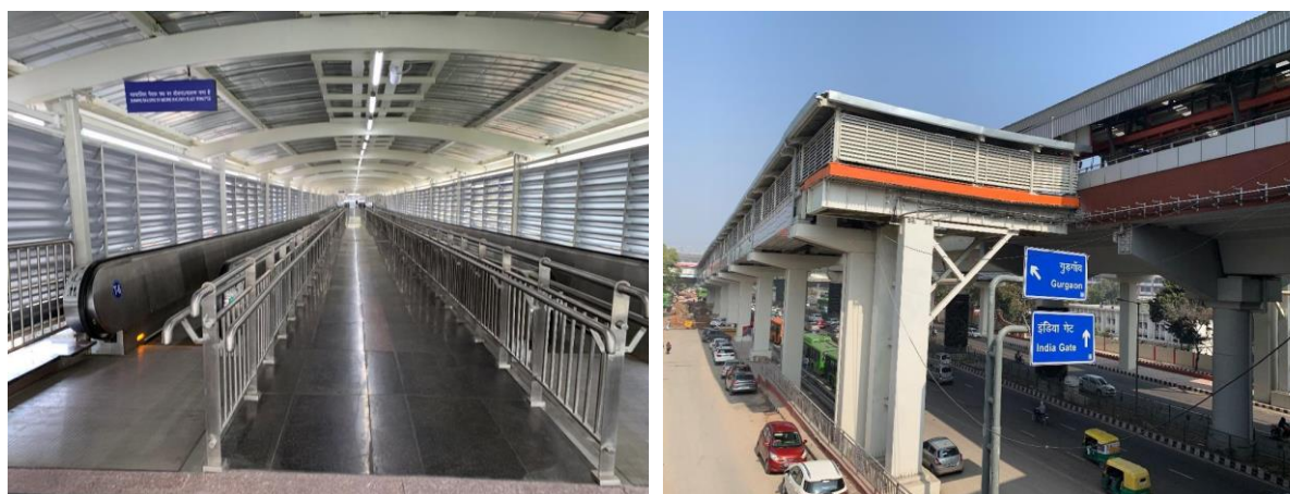
Figure 4-1: A typical skywalk (inner and outer view)
