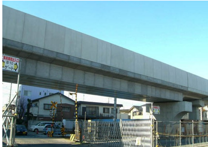
Figure 3-16: Precast Noise Barrier
