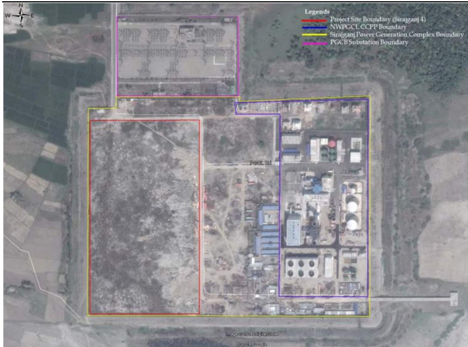
Figure 3.1 Aerial View of the Project Site in Sirajganj Power Generation Complex
