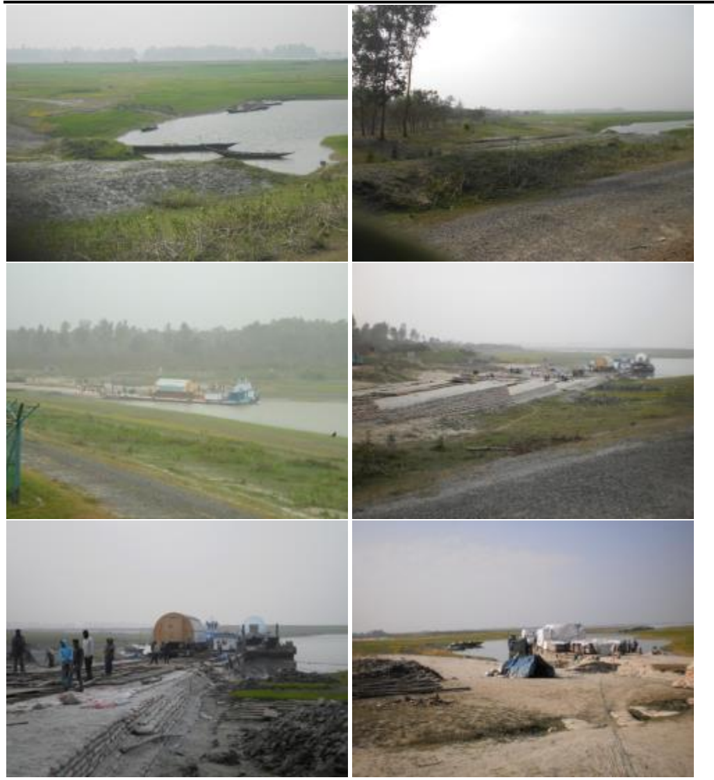
Source: ERM Site Visit (February 2015) and Old Pictures provided by SNWPCL
