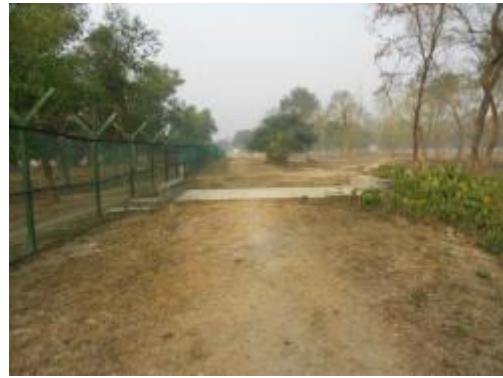
Culvert, BBA Internal Road and Southern Fence
