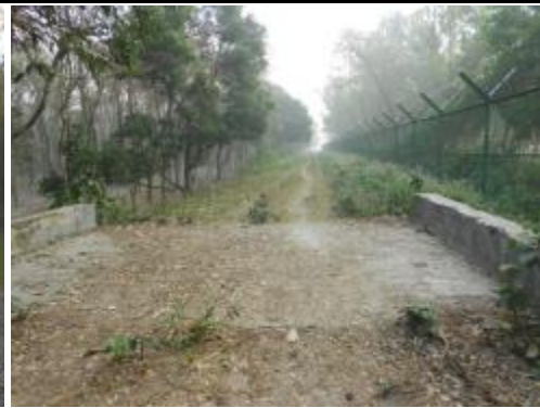
Internal Road Connecting to West Guide Bund
