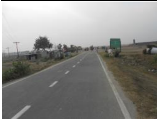
Approach Road connecting National Highway
