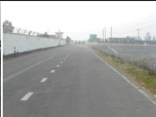
Approach Road near Entrance to Saidabad Power Generation Complex
