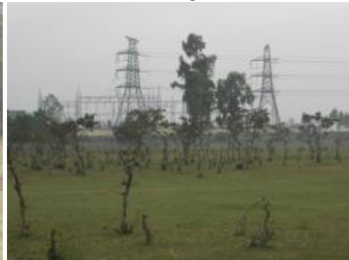
Open BBA Land – North of PGCB Sub-station
