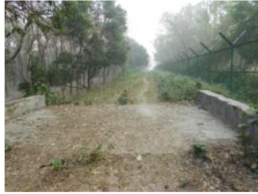
Culvert, BBA Internal Road and Southern Fence
