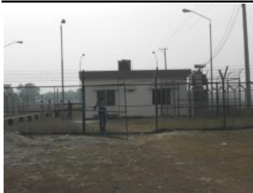
HSD Pumping Station of NWPGL at Bangbandhu Bridge West Railway Station
