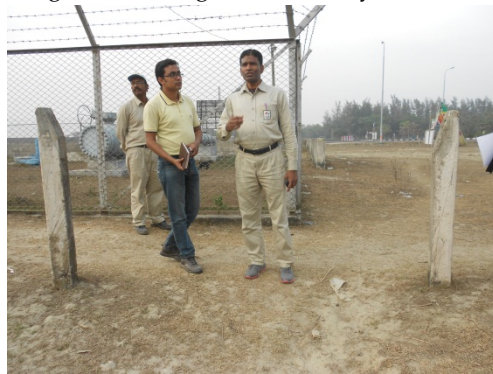
GTCL Valve Station with Pillars indicating Underground Gas Pipeline RoW
