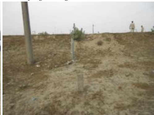
Underground HSD Pipeline Pillar and Cathode Protection
