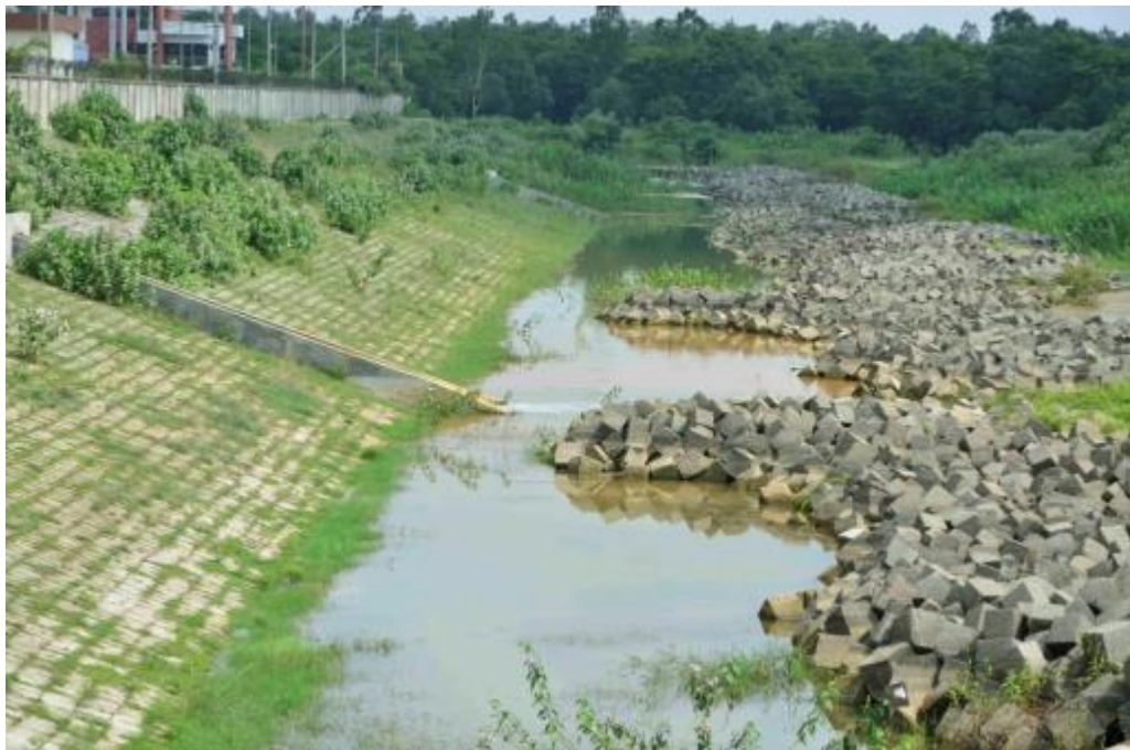
Discharge location of Sirajganj 1 Project
