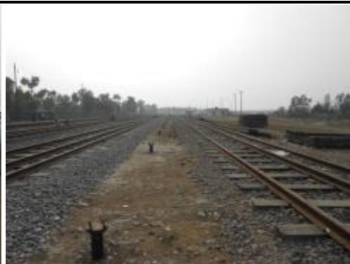
Dedicated Railway Siding of NWPGL and Pumping Arrangement
