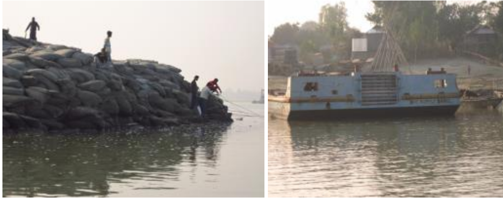
Geobags at various points in the Jamuna River Trawler for carrying dredged sediments
