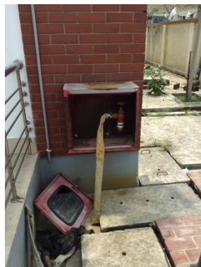
Damaged Hose of Hydrant System in RMS Building
