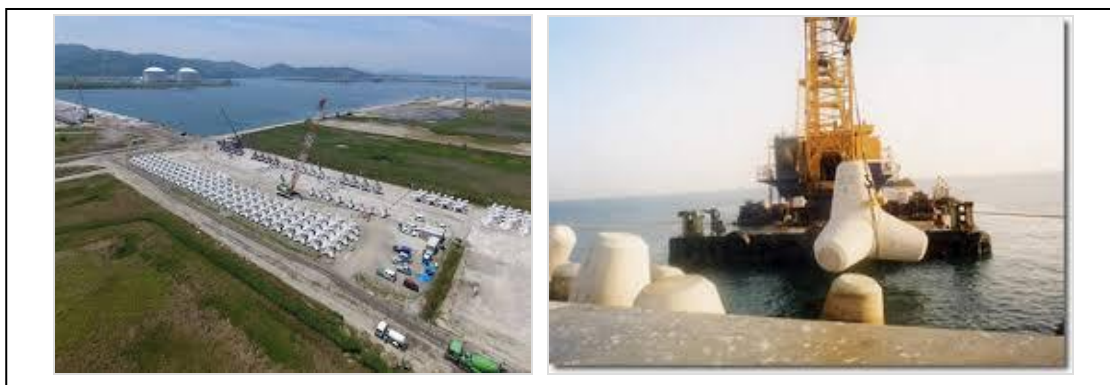
Figure 2.6-11 Sample Picture of fabrication and installation of armor concrete block
