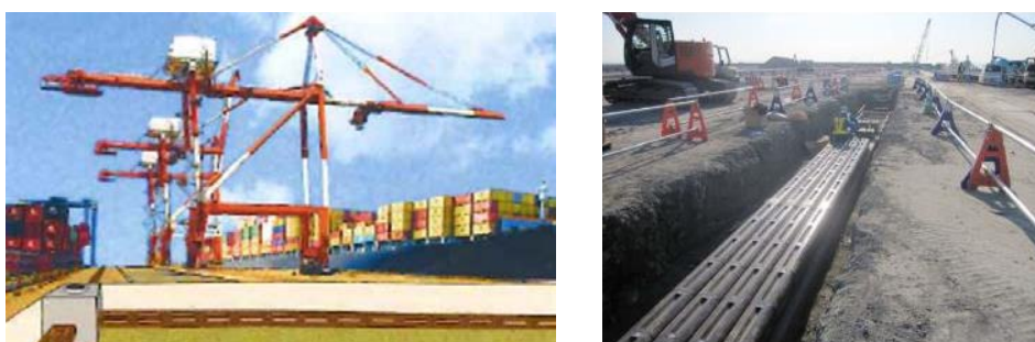
Figure 2.5-45 Example of Cable Duct in a Port in Japan
