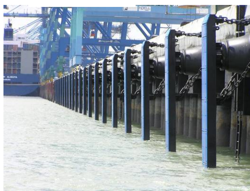
Figure 2.5-5 Rubber Fender System
