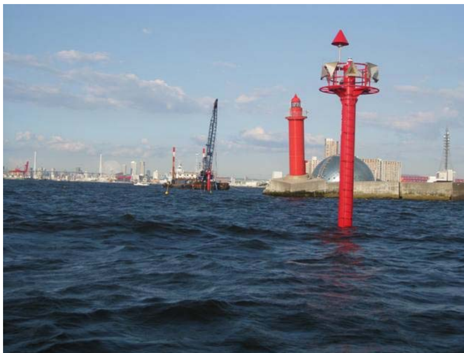
Figure 2.5-35 Pillar-type Lighted Buoy
