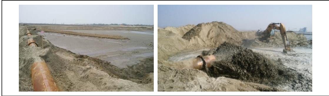
Figure 2.6-7 Sample Picture of on-shore disposal method
