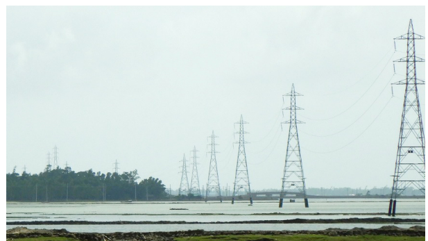
CPGCBL's Power Line (132 kV)
