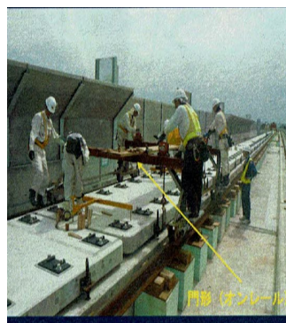
Laying the concrete slab
