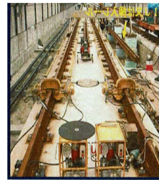
Rail Setting and installation of insulation joint
