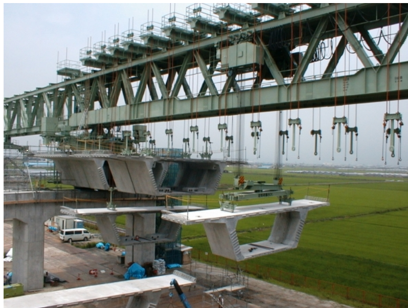
Figure 4.5.37 The Span by Span Method Girder Erection
