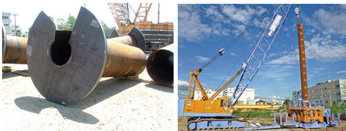
Figure 4.15.3 Screw Steel Pipe Piles
