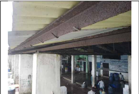
Photo 1-5: Tops of columns at Fish Handling Shed B
