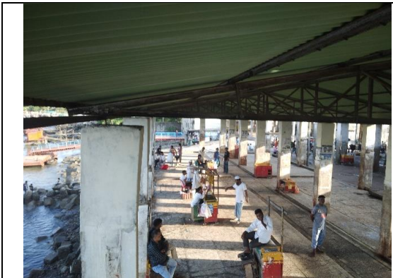
Photo 1-4 : Tops of columns at Fish Handling Shed A
