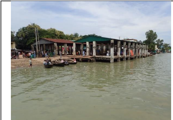
Photo 1-6 : Front side of the fish handling shed (at high tide)
