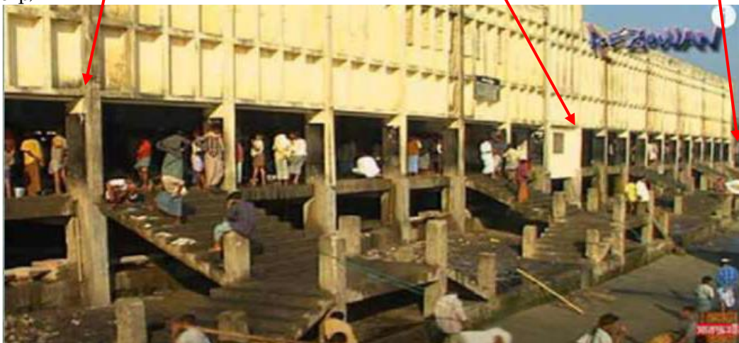
Photo 1-3 : The stairway jetties in front of the existing fish handling shed before the collapse
