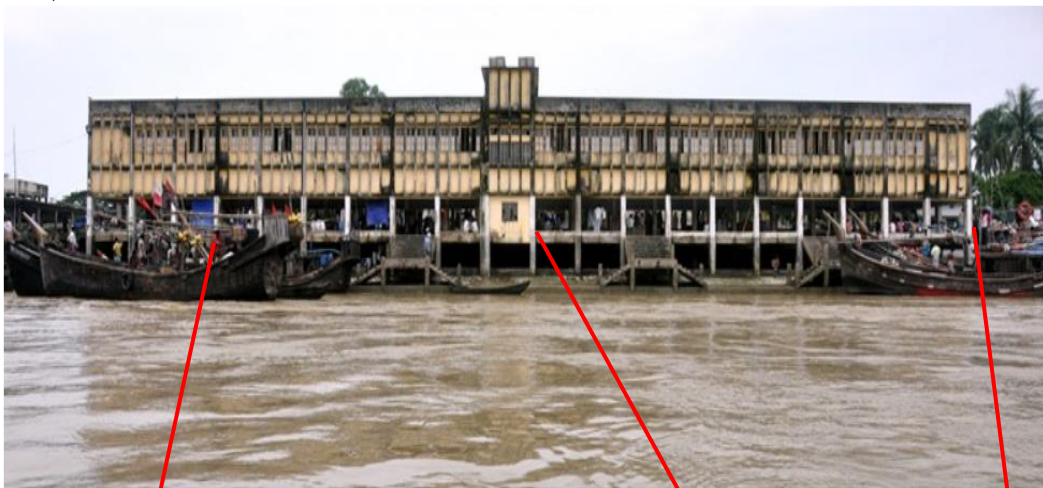
Photo 1-2 : The fish handling shed before it collapsed (Source: Flickr.com Author: rony_crp)
