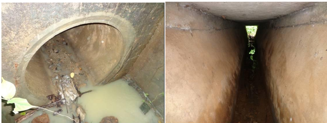
Photo 2.1 Existing Pipe Culvert (L) and Slab Culvert (R) Along NH51
