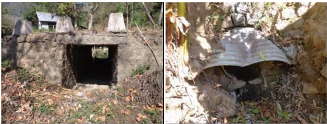
Photo 2.1 Existing Slab Culvert (L) and GI Sheet (R) Along NH54
