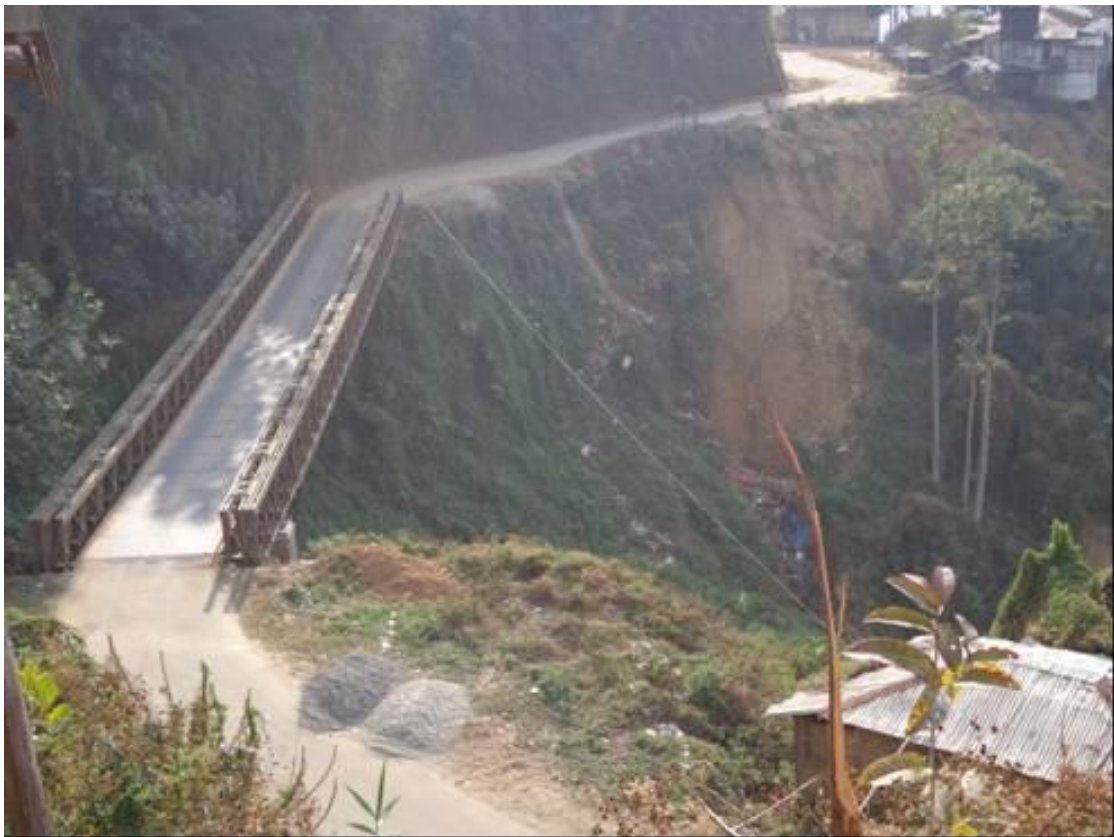
Figure 7.2.1 Temporary Bridge at Chhingchip at 74+660
