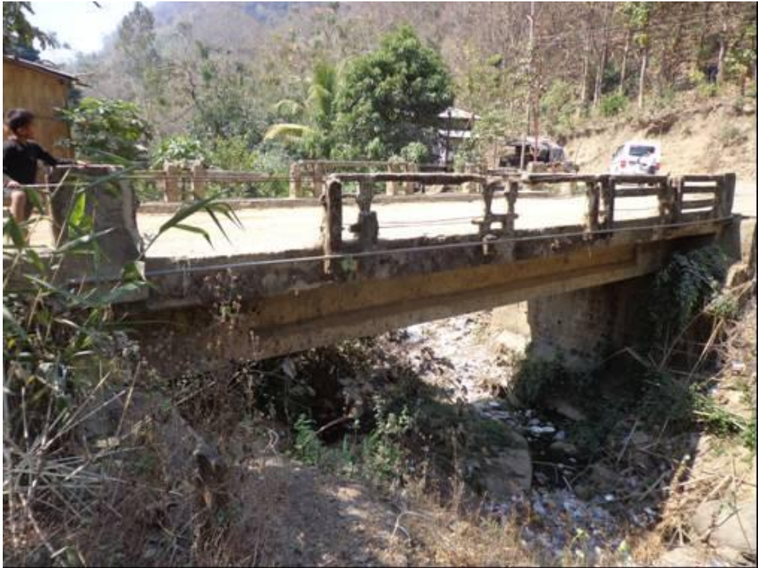
Figure 7.2.2 RC T beam Bridge at Maudarh at 190+190
