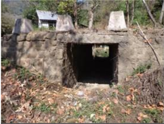
Figure 7.2.17 An example of existing slab culvert
