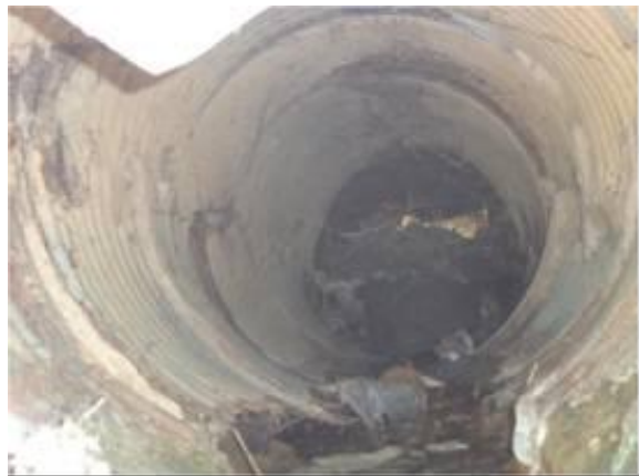
Figure 7.2.19 An example of existing G.C.I. Sheet pipe
