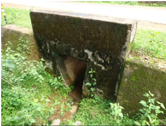
Figure 8.2.9 An example of existing slab culvert (narrow inner width)
