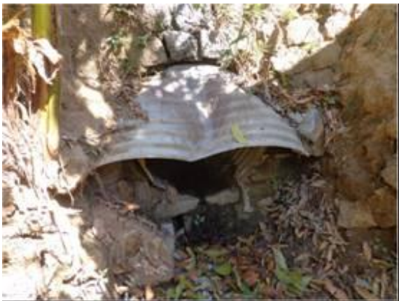
Figure 7.2.19 An example of existing G.C.I. Sheet pipe
