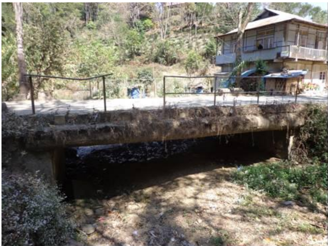
Figure 7.2.3 Slab Bridge at Zobawk at 216+450
