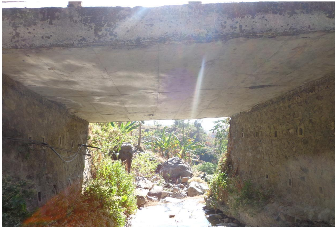
Figure 7.2.20 An example of existing large slab culvert
