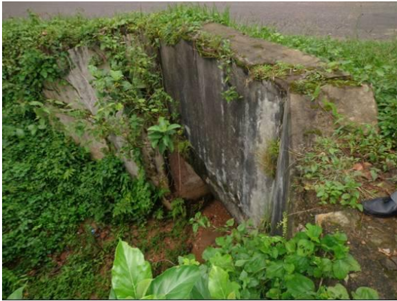
Figure 8.2.8 An example of existing slab culvert
