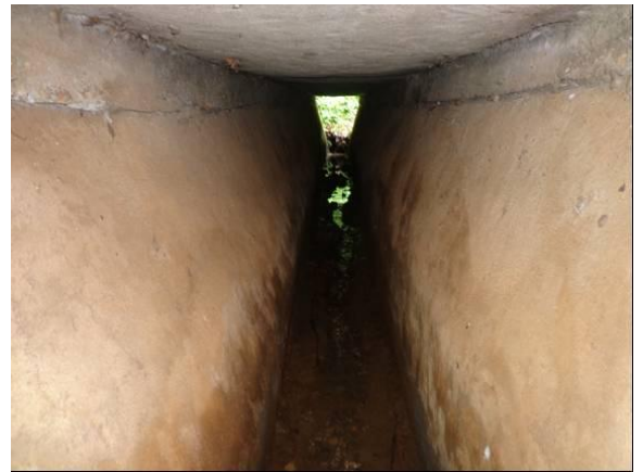
Figure 8.2.9 An example of existing slab culvert (narrow inner width)
