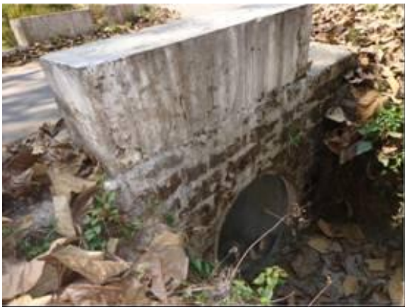
Figure 7.2.18 An example of existing R.C. Hume pipe
