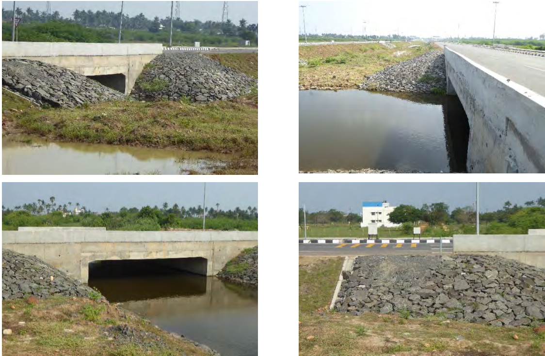
図 6.2.55 BoxCulvert (Outer Ring Road)
