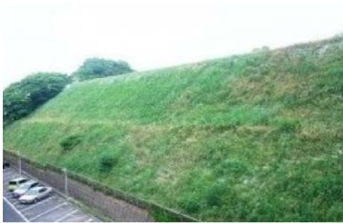
Planting slope protection method
