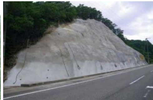
Mortar Spraying slope protection method
