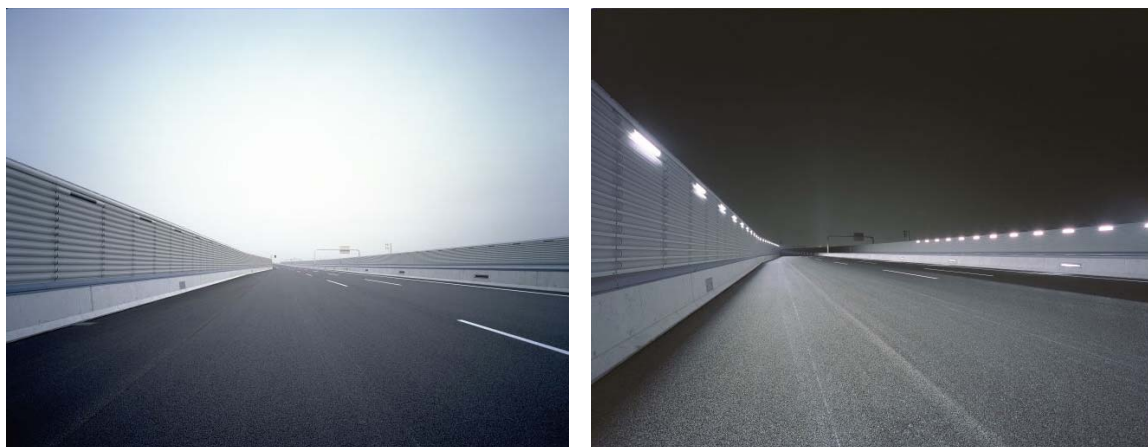
Figure 6.2.9 Noise Barrier with Lighting System in the handrail/noise barrier/view barrier
