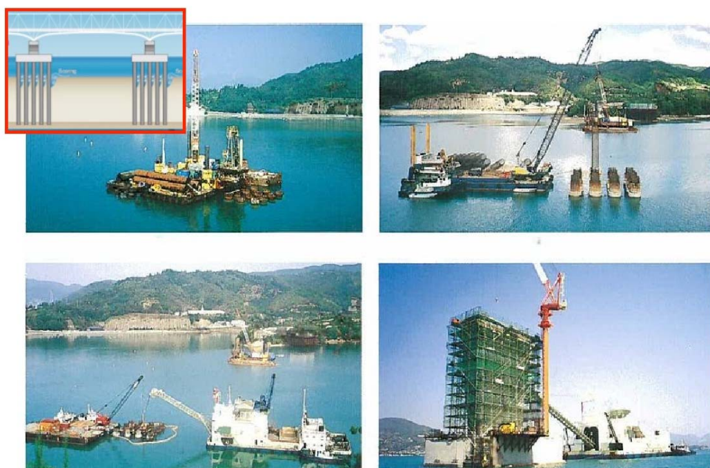
Figure 6.1.6 Bored Piling Methodology for Pollution Control
