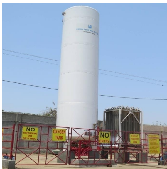
Photo 2g: LOX Storage Facility on Plot
