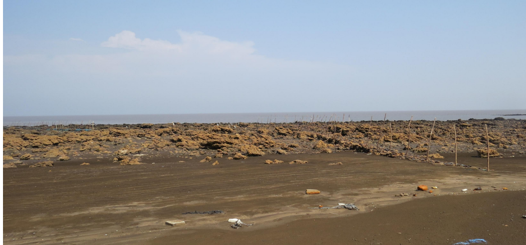
Photo 5.h: Site Selected for Dry-dock 2 (as in April, 2015)
