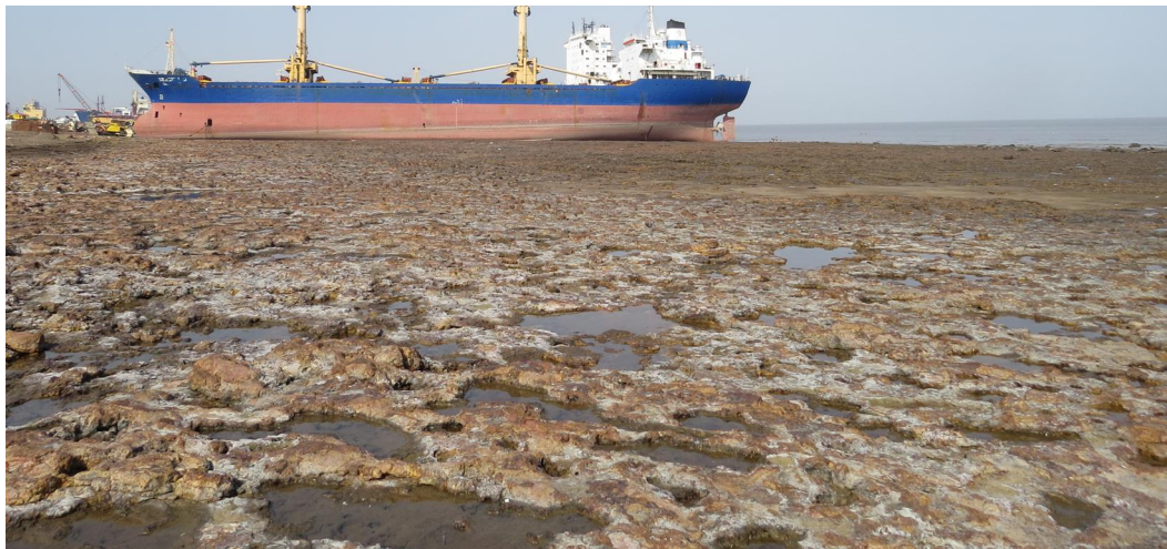
Photo 5.g: Site Selected for Dry-dock 1 (As in April, 2015)
