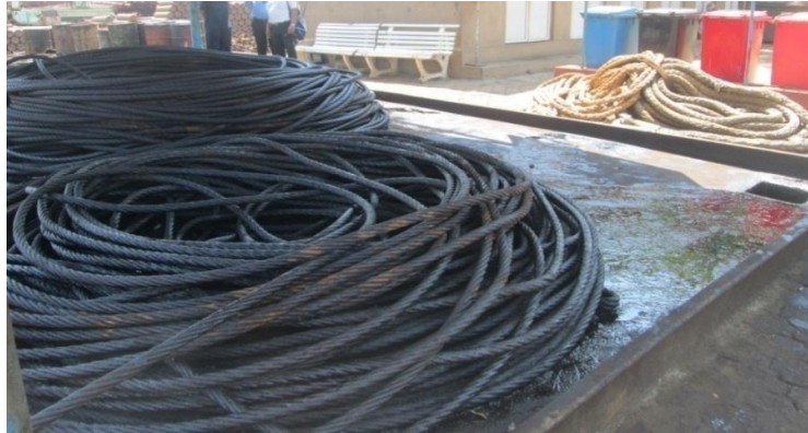
Photo 4.j: Oily Cables Stacked Properly
