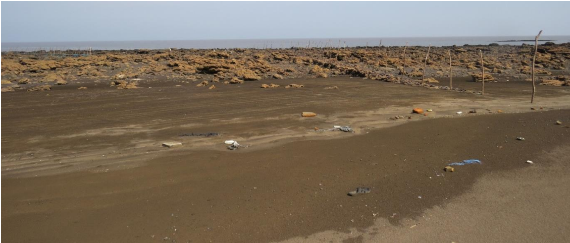
Photo 2.b: Proposed Site of Dry Dock 2 as in April, 2015
