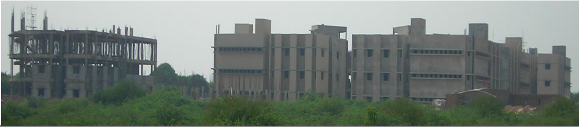
Photo 2.f(ii): Under Construction Workers' Barracks as in Oct., 2015
