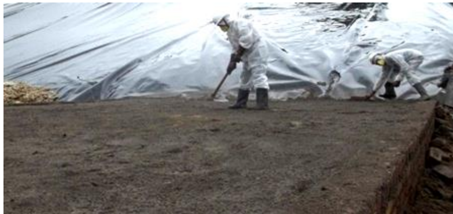
Photo 4.h: ACWM being Cemented Over
