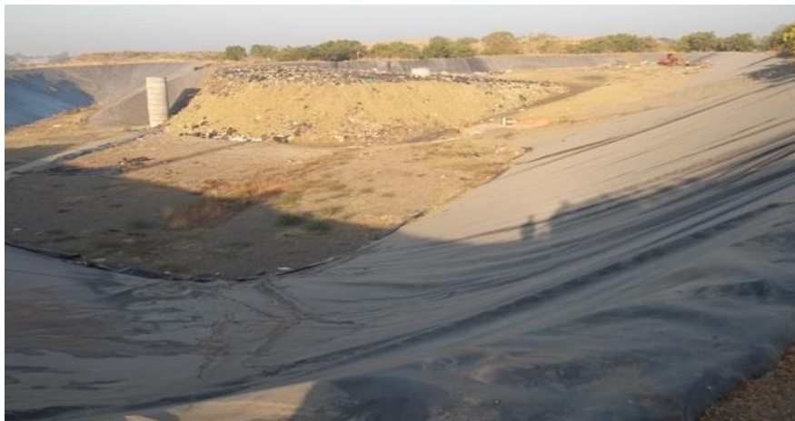
Photo 4.j: Operational Hazardous waste Disposal Land-fill
