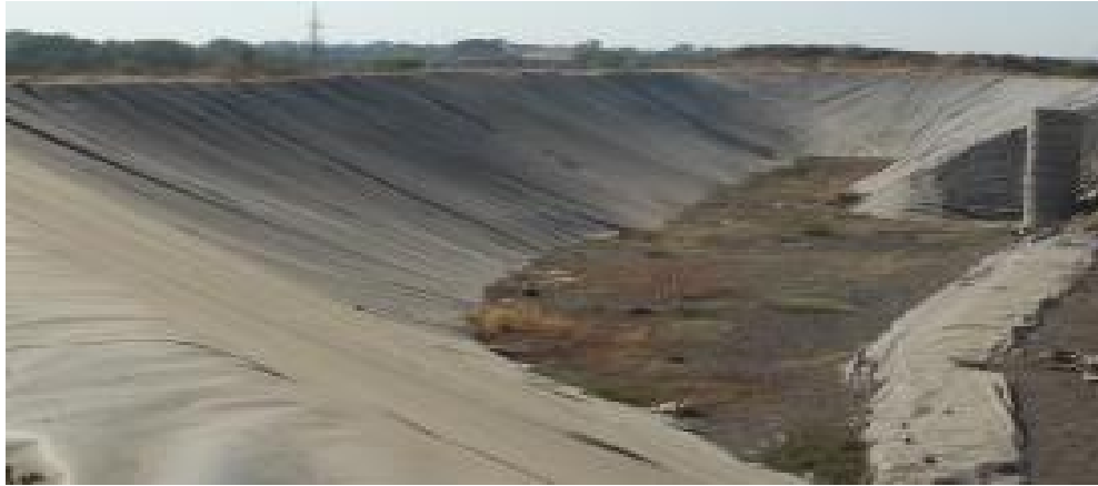
Photo 4.k: Newly Built MSW Landfill
