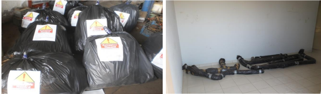
Photo 4.e: Asbestos & ACM stored Prior to Final Disposal
