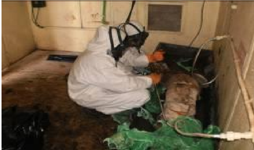
Photo 4.d: Workers Engaged in Asbestos Removal
