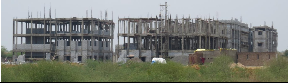
Photo 2.f(i): Under Construction Workers' Barracks as in April, 2015
