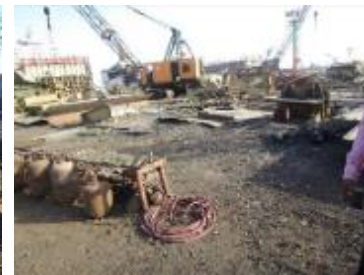
LPG is stored close to cutting zone (Normal yards)
