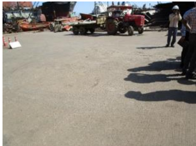
Concrete floor on the yard (NK certified yard)
