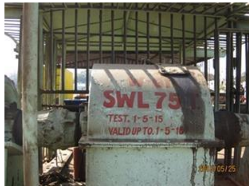
P.19 75 t Winch with fence
