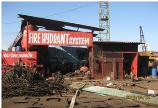
P.36 Fire Station
