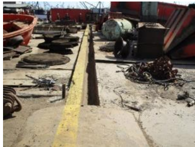
Drainage pit to prevent pollution on the soil and sea (NK certified yard)
