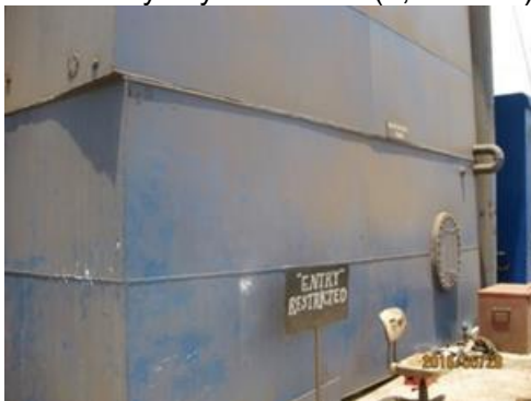
P.V-7 Bilge water tank (45,000 liter)
