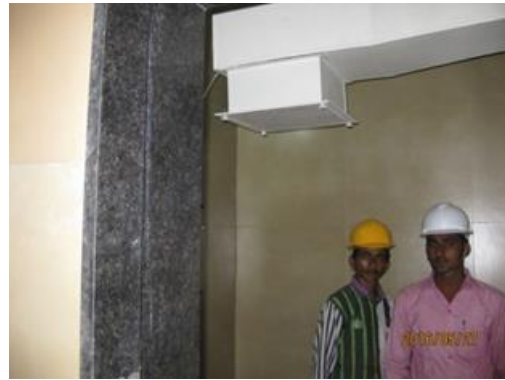
P.V-5 inside of negative pressure chamber
