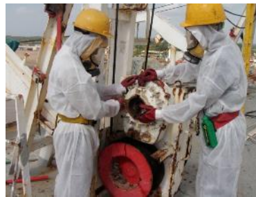
Asbestos removal on board (NK certified yard)
