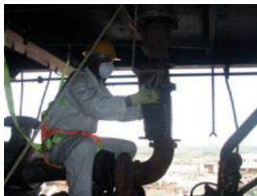
Wearing safety belt during working at height (NK certified yard)
