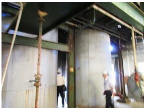
Capacity 7,000 KL/year Product Tank after 1 st distillation
