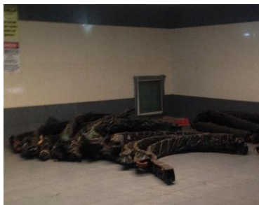
Asbestos contained parts are sealed and stored (NK yard)
