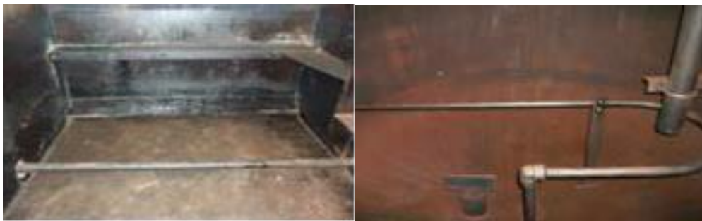
Figure 11-29 Image of fuel tank before and after cleaning by MDS
