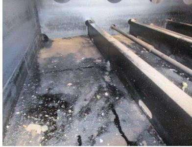
Oil still remaining inside fuel tank after cleaning (yard in process of verification)
