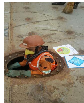
Entry after safe for entry procedure confirming the label (yard in process of verification)
