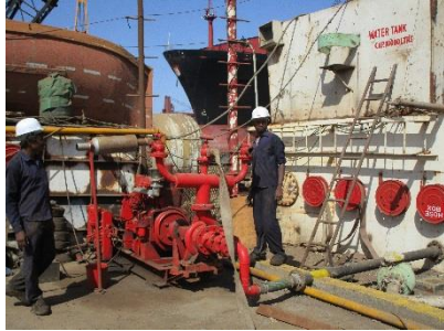
Fire fighting facility (Normal yards)
