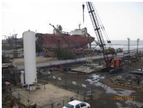
P.30 liquid oxygen tank
