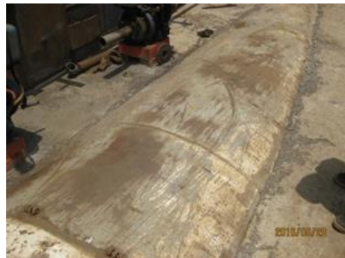
P.V-7 Rain Water tank (15,000 liter)
