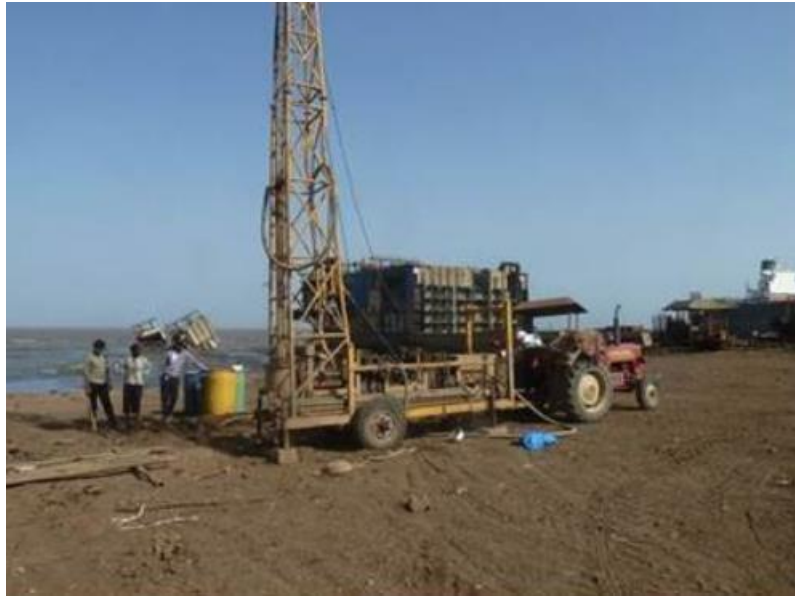
Figure 3-5 Boring at Seashore
