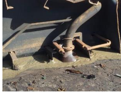
Water coming inside the fuel tank while the ship is waiting in inter-tidal zone (yard in process of verification)
