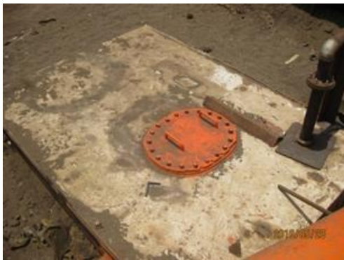
P.V-7 Dirty oily water tank(5,000 liter)
