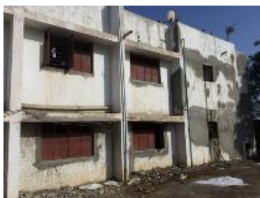
Dormitory provided by ship recycling yards
