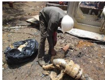
No gloves during glass wool removal (Normal yards)
