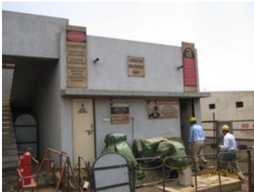
P.V-5 entrance of negative pressure chamber
