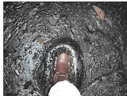
Sludge before cleaning
