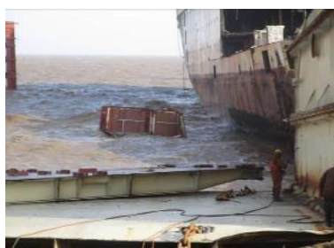
Blocks being dropped in the sea / in the inter-tidal zone (Normal yards)
