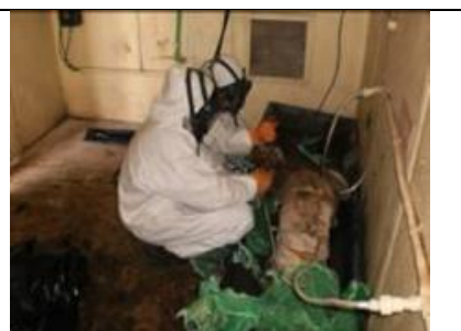
Asbestos removal by mobile decontamination unit (All yards)
