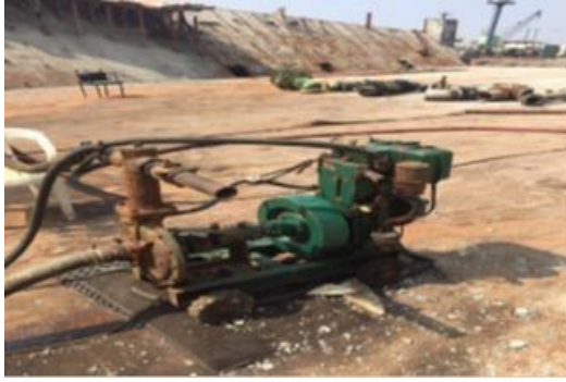
P.V-7 Mobile fire pump onboard
