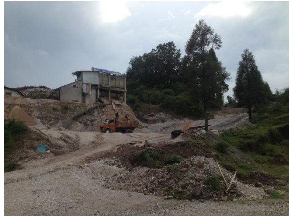
Pic. 7 Hill-cutting/ stone crushing near Umtyngar
