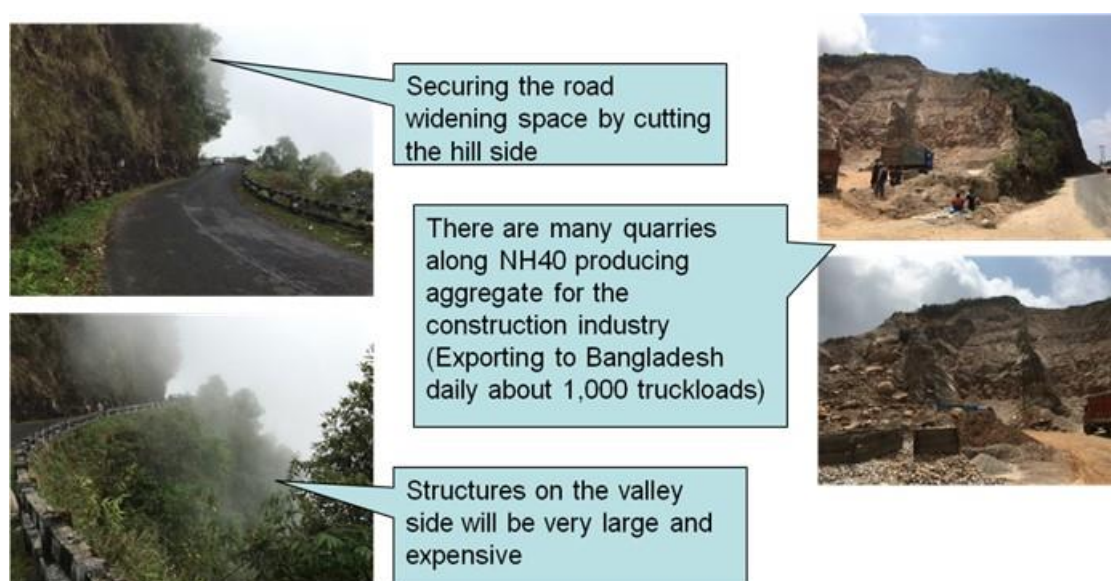
Figure 3-26: Road Widening of Cliff Sections
