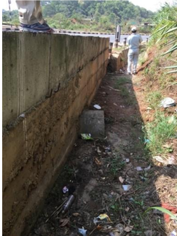
Figure 5-79: Accumulated Earth in Drainage
