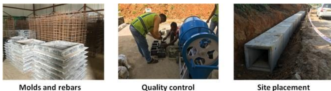
Figure 3-25: Example of Adoption of Concrete Precast Method
