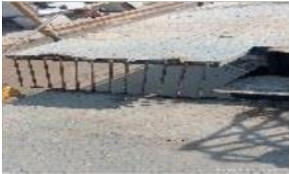
Mesh is made to cover gaps between bulkhead and shutter
