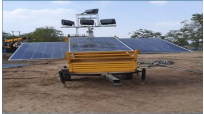
Use of Solar lights at C4 package
