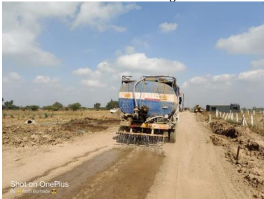
Water sprinkling at chainage 188
