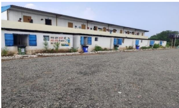
Good housekeeping and vegetation at labour Camp at Ch 321, Sec-04, C4 Package
