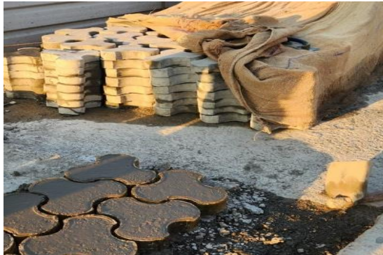
Concrete tiles made from C&D Waste in C6 package. Tiles will be reused in the Project site area
