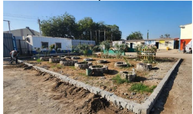
Planters made out of waste concrete blocks at Ch 407 in C6 package
