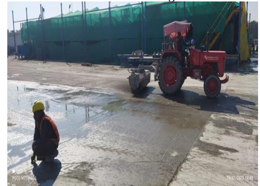
Mechanical mopper at chainage 188
