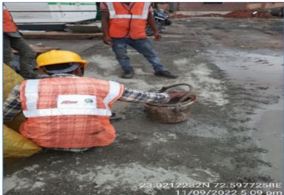
Waste cement, concrete & concrete blocks reused at site level for different purpose like potholes repairing, placing on barricading boards for protection, Concrete block making, etc. and Used Concrete block (QC lab) reused for wall preparation, etc at C7 Package
