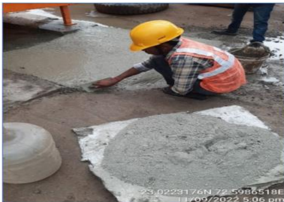
Waste cement, concrete & concrete blocks reused at site level for different purpose like potholes repairing, placing on barricading boards for protection, Concrete block making, etc. and Used Concrete block (QC lab) reused for wall preparation, etc at C7 Package
