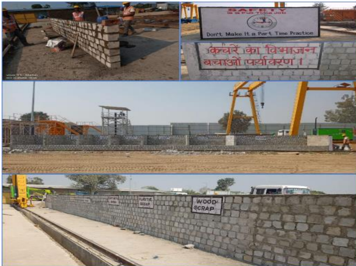
Used concrete blocks reused for scrap yard development at Casting yard at C7 Package
