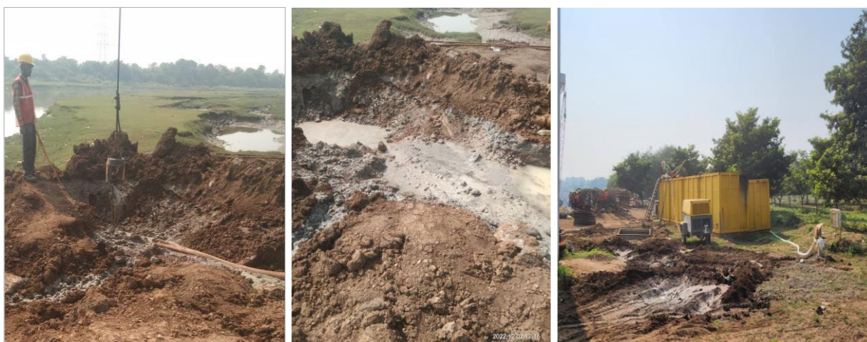
Figure 48: Pit after Pumping of Polymer to De-sanding container
