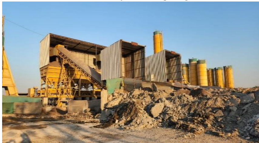
Dust control measures adopted at Batching plant in C6 package
